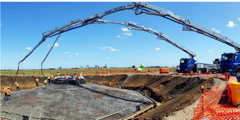
FIGURE 2-2 TYPICAL FOUNDATION BEING CONSTRUCTED
