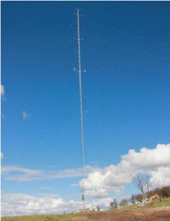
FIGURE 2-10 TYPICAL METEOROLOGICAL MONITORING MAST
