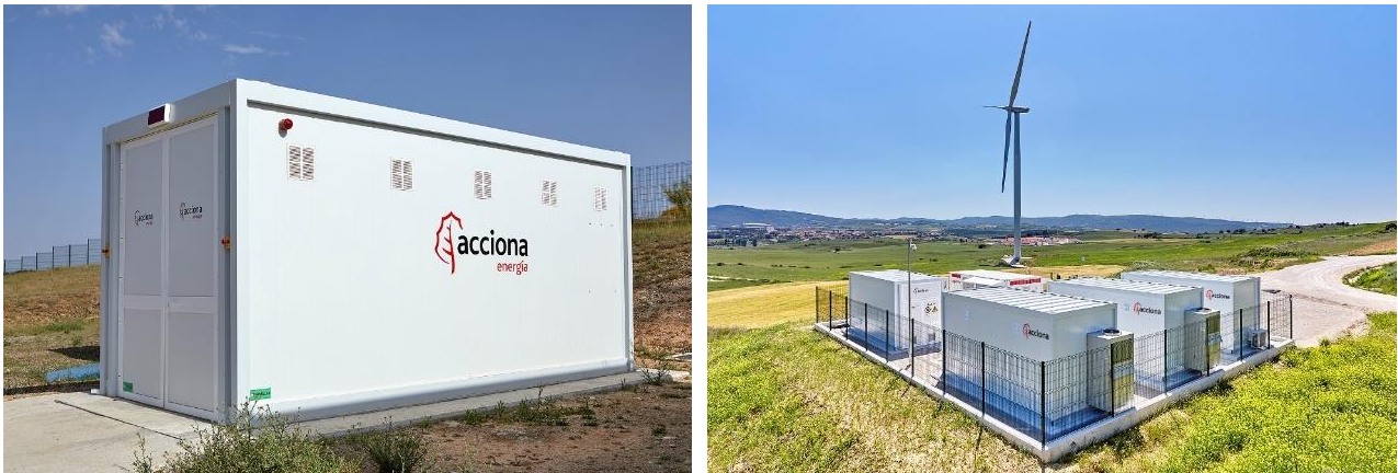
FIGURE 2-8 TYPICAL 200 MW/800 MWH BATTERY ENERGY STORAGE SYSTEM
