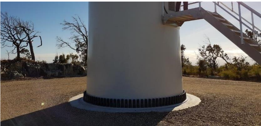
FIGURE 2-3 TYPICAL FOUNDATION POST-CONSTRUCTION
