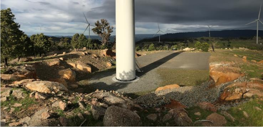
FIGURE 2-4 TYPICAL HARDSTAND AREA
