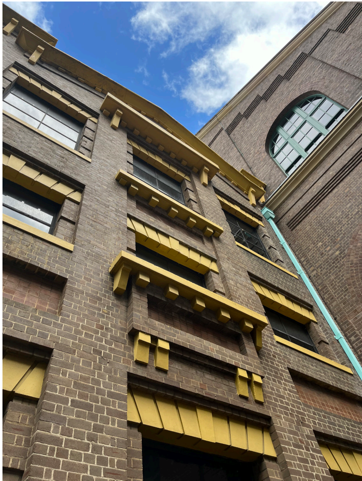
Switch House - Brick and Rendered lintels
