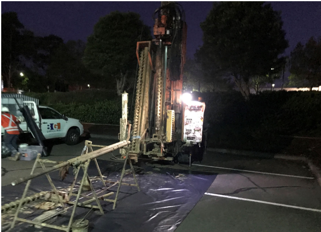
Photo 4 - Setting up the drilling rig -Hanjin D8
