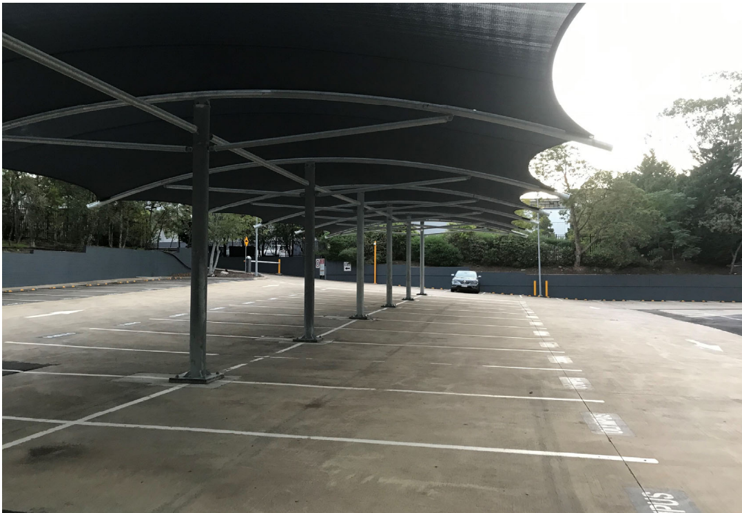
Photo 3 - Carpark areas in the north of the site looking north-east
