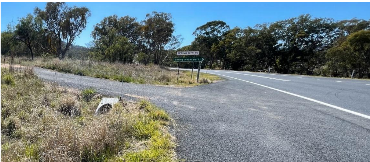
Plate 4.2 Existing fingerboard sign on the eastbound approach to the Gwydir Highway/Spring Mountain Road intersection
