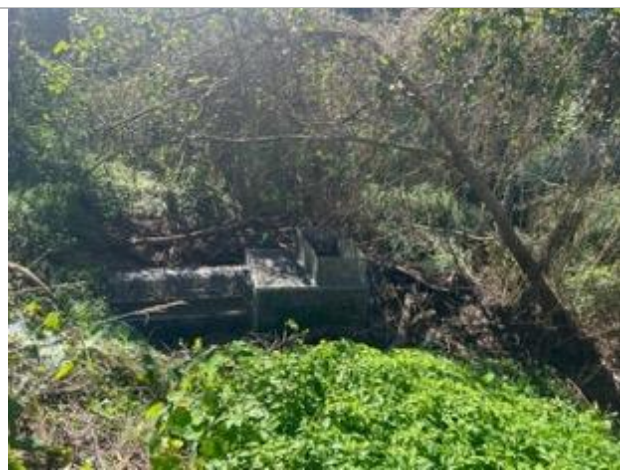
Plate 2. Area near existing GPT to be regraded and planted and to have adaptor to take water and disperse it along the slope prior to going into the creek.
