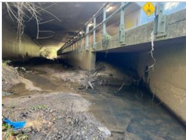
Plate 4. Sediment removal upstream is recommended. A Barami or similar can be used to divert sediment out of the creek and into a park-land area that is currently weed dominated. Materials can be used within the site to suppress weeds and then replant with natives.
