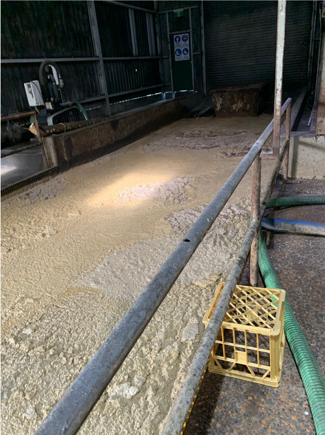
Photo 1. Sludge tank extension
