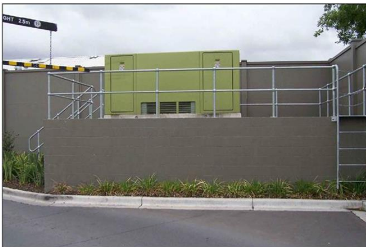
Figure 51 - Example substation raised above 1:100 flood level
