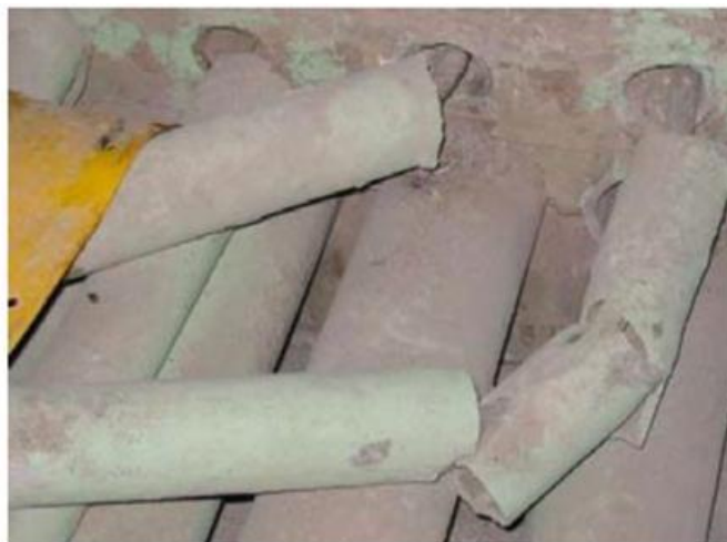
The picture may let someone know if they find this while digging they are dealing with a hazard. This is an example of ACM cable ducts found in Endeavour Energy's electricity network during excavation for underground works.
