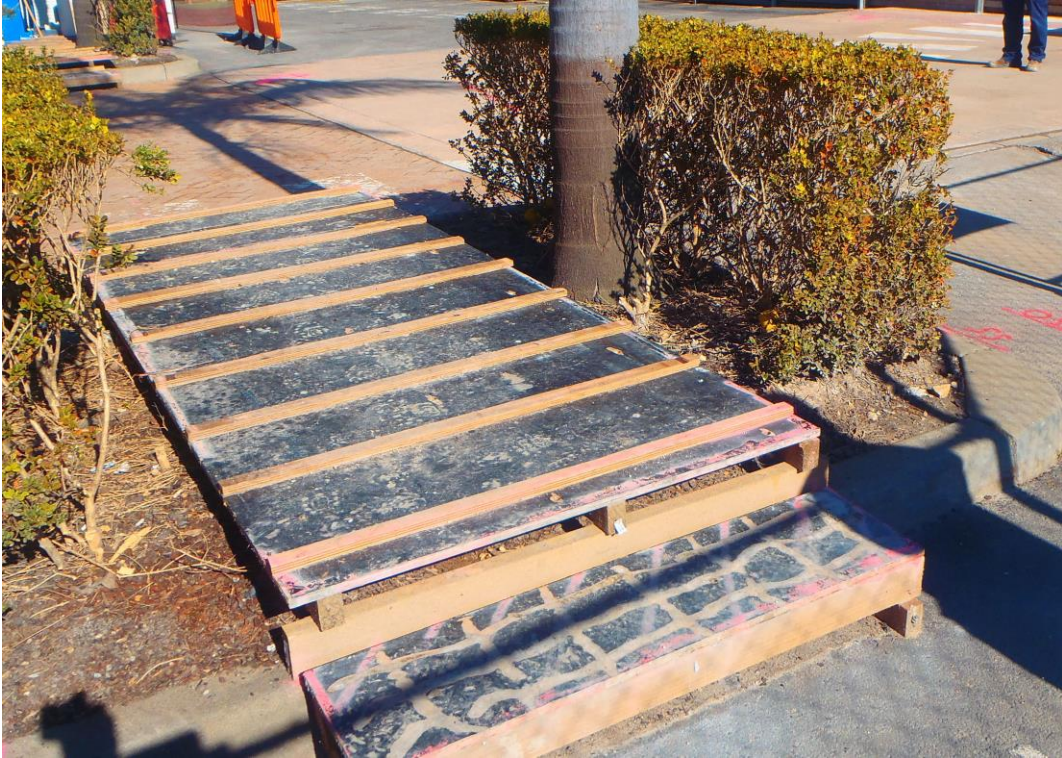
Plate A: An example of board protection to reduce compaction over the root zone. This technique should be used over the root zone of Trees 1, 2, 3 and 6. P. Vezgoff.
