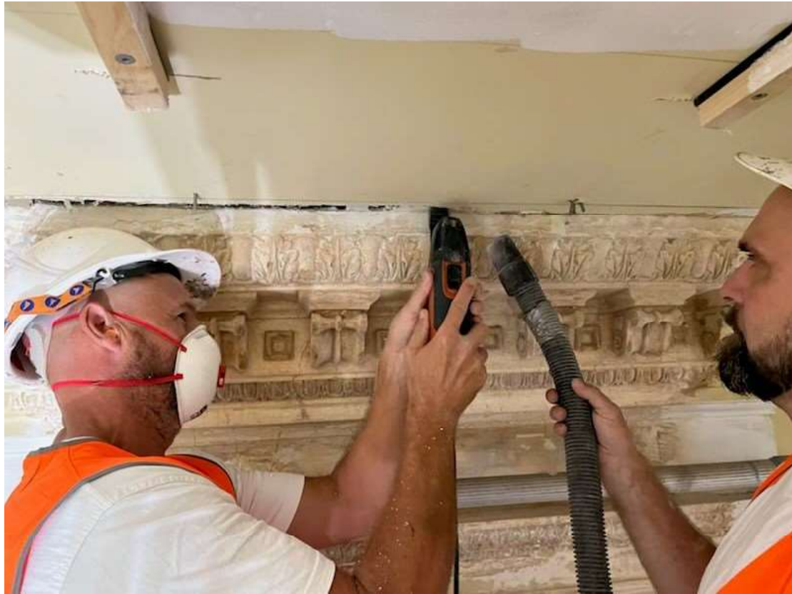
IMAGE 1.4 – Oscillating cutter being used to cut through timber lathes
