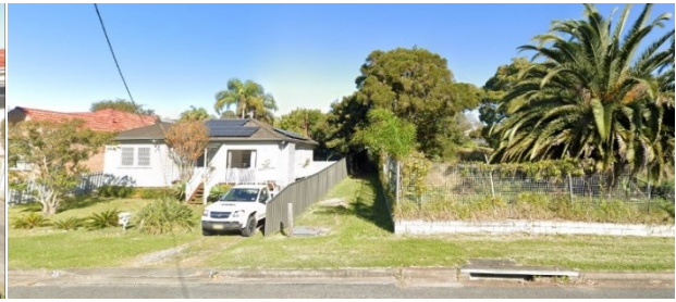
Figure 6 Informal pedestrian accessway looking south from James Street
