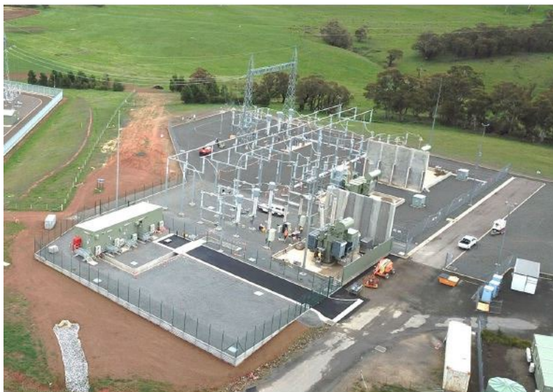
Figure 3-15 Typical Substation - Gullen Range Wind Farm 33/330kV Substation
