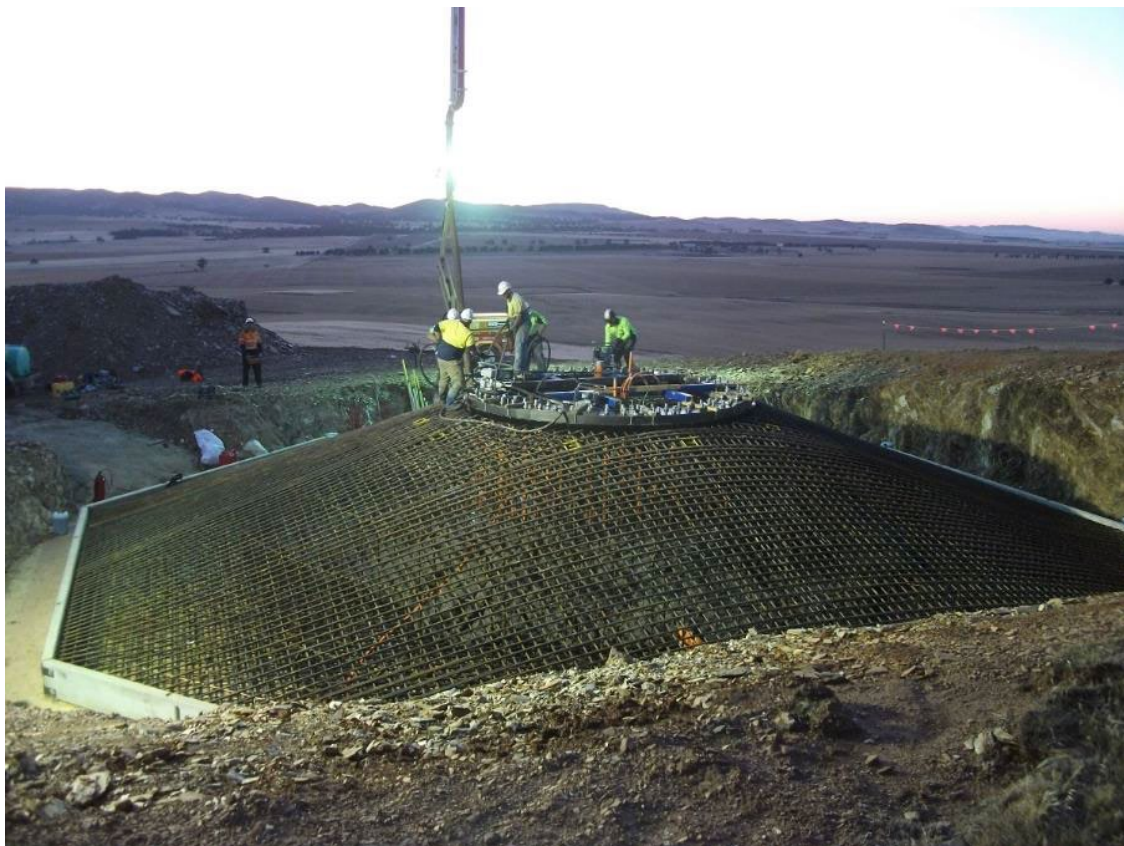
Figure 3-11 Typical Gravity Foundation for a Wind Farm (ENGIE Willogoleche Wind Farm in construction)
