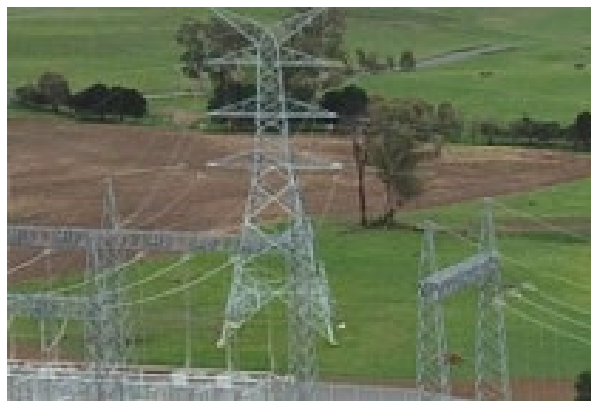
Figure 3-14 Typical 330 kV Lattice Tower
