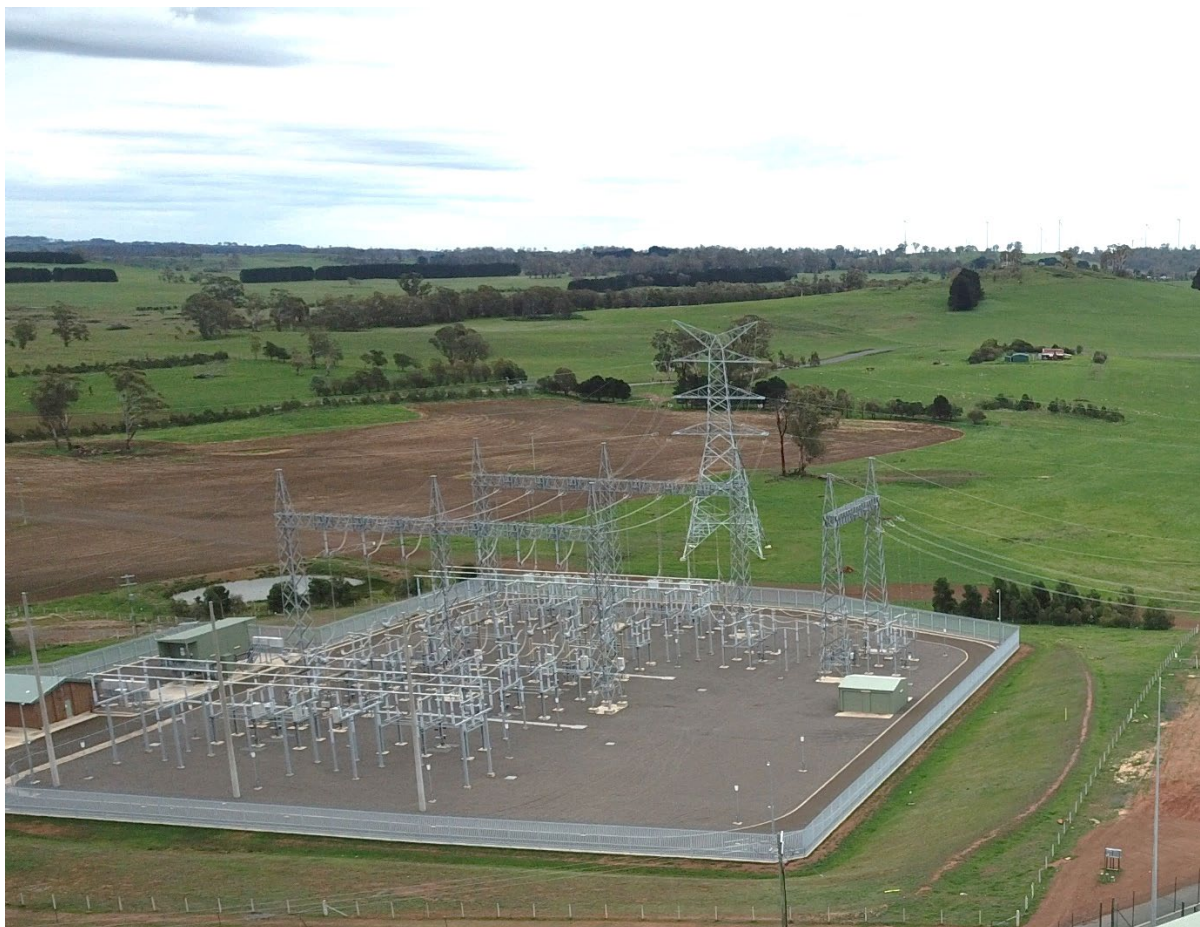
Figure 3-17 Typical Switching Station – Gullen Range Wind Farm 330 kV Switching Station
