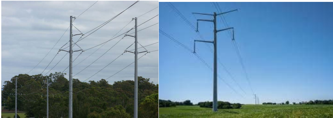
Figure 3-13 Typical Steel Pole Structures, Transmission Line
