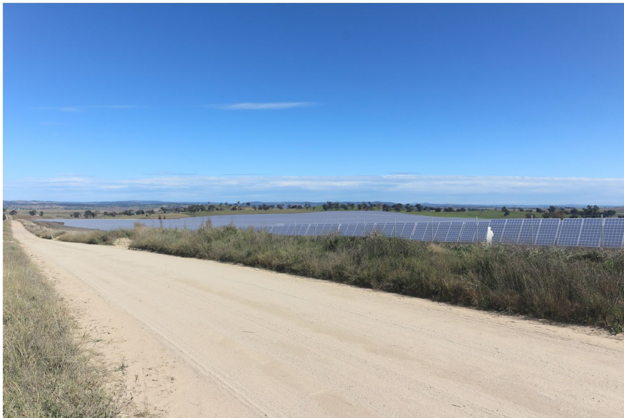
Figure 5-2 View south along Brewongle Lane, photomontage (day 1, no planting shown) (Source: Iris)
