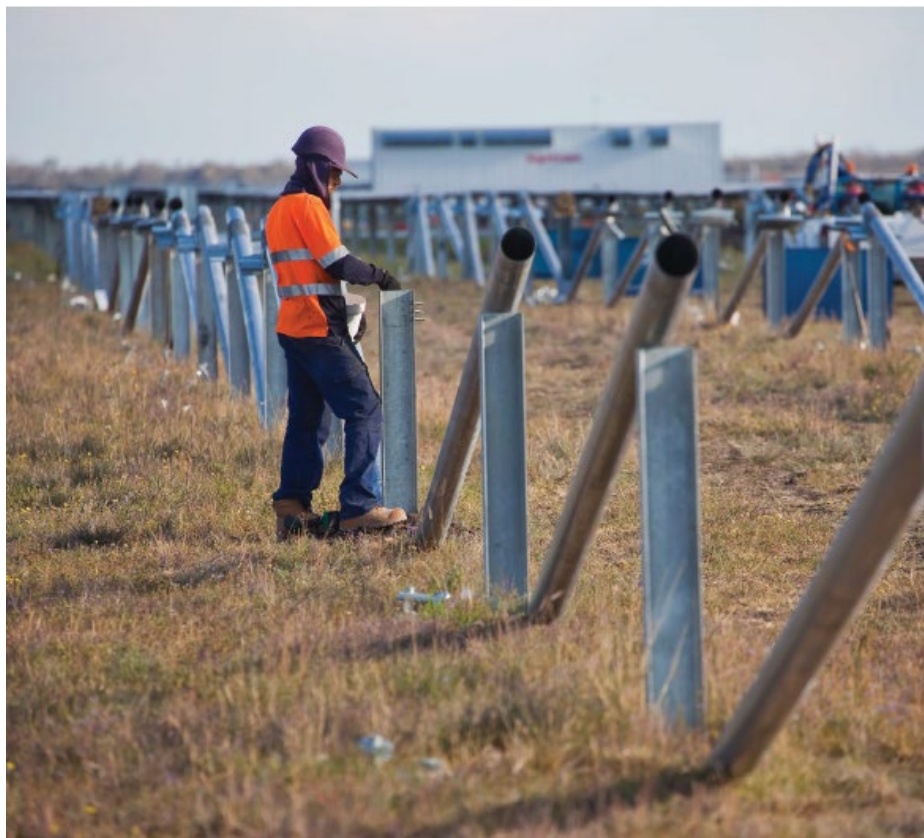
Figure 4-4 Soil disturbance during construction, showing the soil profile and pasture remains largely unaffected (source DPE 2022)
