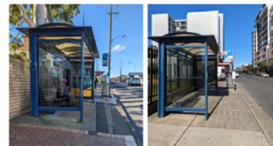
Figure 7-3 No TGSIs (both) and poor surface (left)
