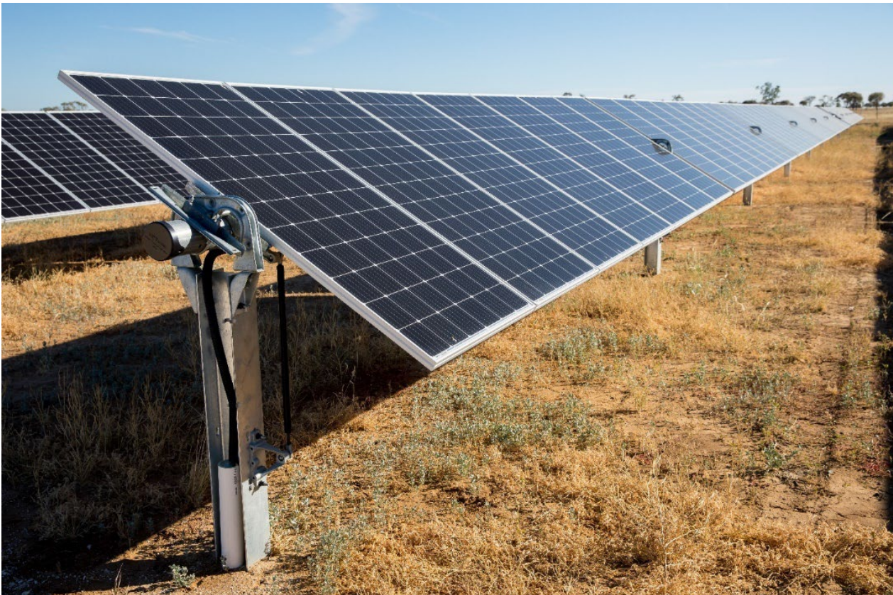
Photograph A.1 PV module row with single axis tracking technology
