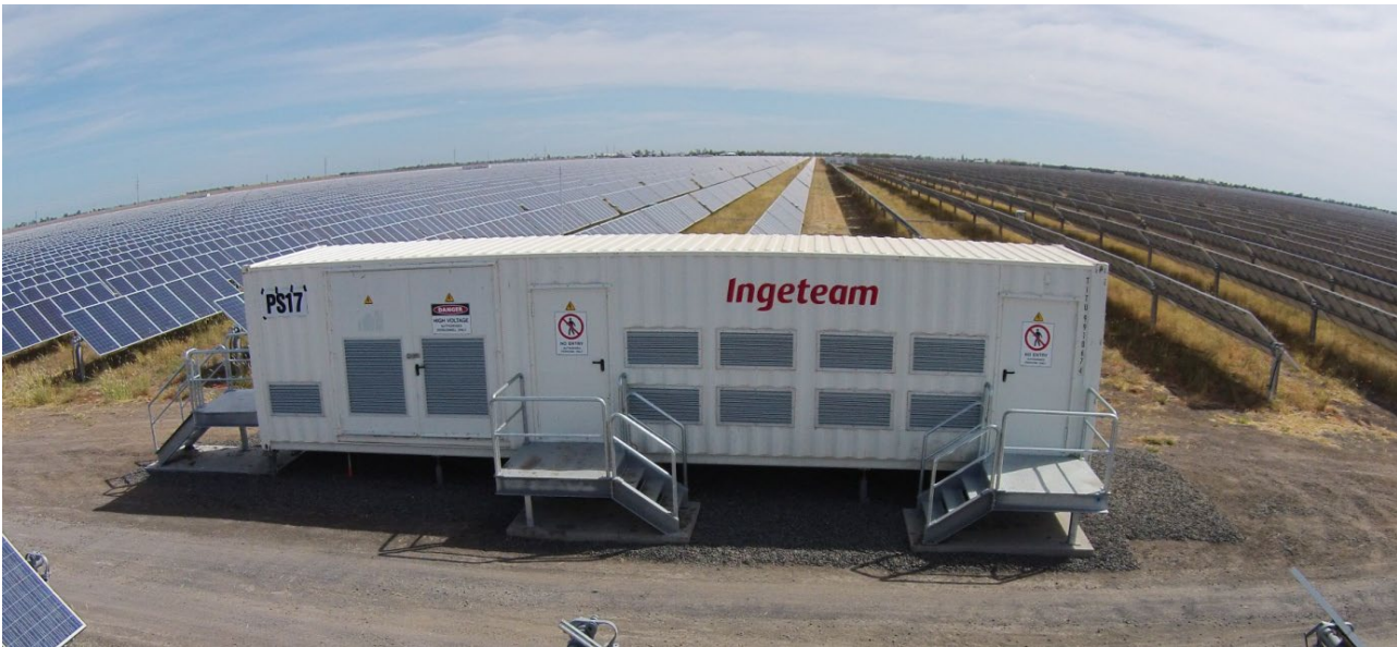
Photograph A.2 Containerised inverter solution with PV module rows
