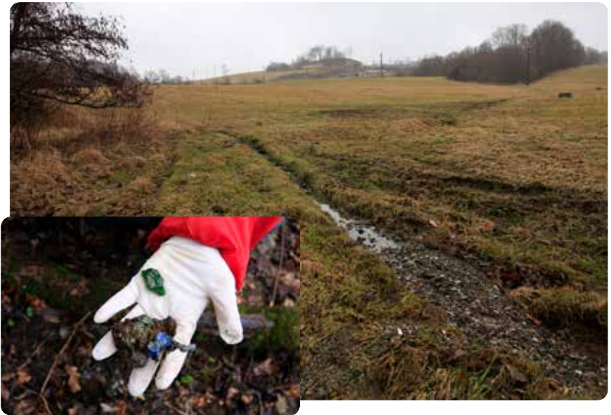
Figure 2: This location is close to the Czech/Polish borders, where mixed fly and bottom ash from MWI was used for the cover layer of landfill (on the top of hill at this photo) and also to fill in the drainage line down the hill through the cattle pasture ending in a nearby creek. Levels of PCDD/Fs measured in the material were up to 0.08 ng TEQ g -1 d.m. Photo: Jan Losenický, Arnika, November 2011.
