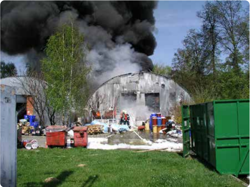
Figure 5: Storage of waste incineration ashes on fire in a hazardous waste incinerator Vyškov, Czech Republic in May 2005. Photo by South Moravian Fire Brigade.
