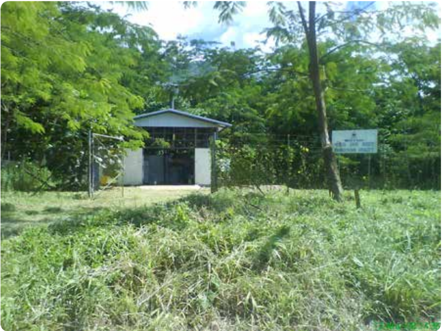
Figure 18: Small medical waste incinerator at Samoa. Photo by Lee Bell.
