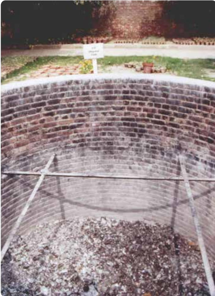
Figure 19: Ash pit in the garden of one of small medical waste incinerators in Lahore as it was in 2005 (see also Annex 16.4). Photo by Jindrich Petrlik, Arnika, March 2005.
