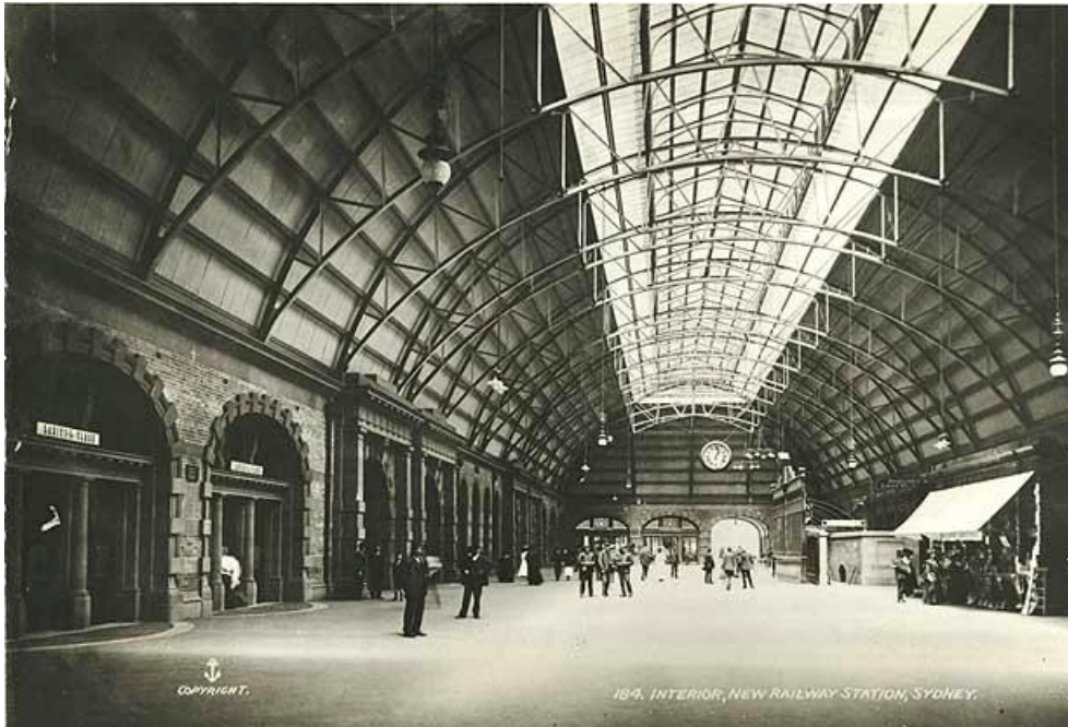
Figure 131. c.1906 Assembly Platform (now known as Grand Concourse) at Central Station. Note the original skylight to the roof and glass pavement lights to the door thresholds. 401
