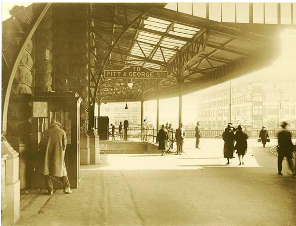
Figure 132. c.1924 Porte-Cochere. Note the skylights to the roof, glazed valances and pavement lights. 402
