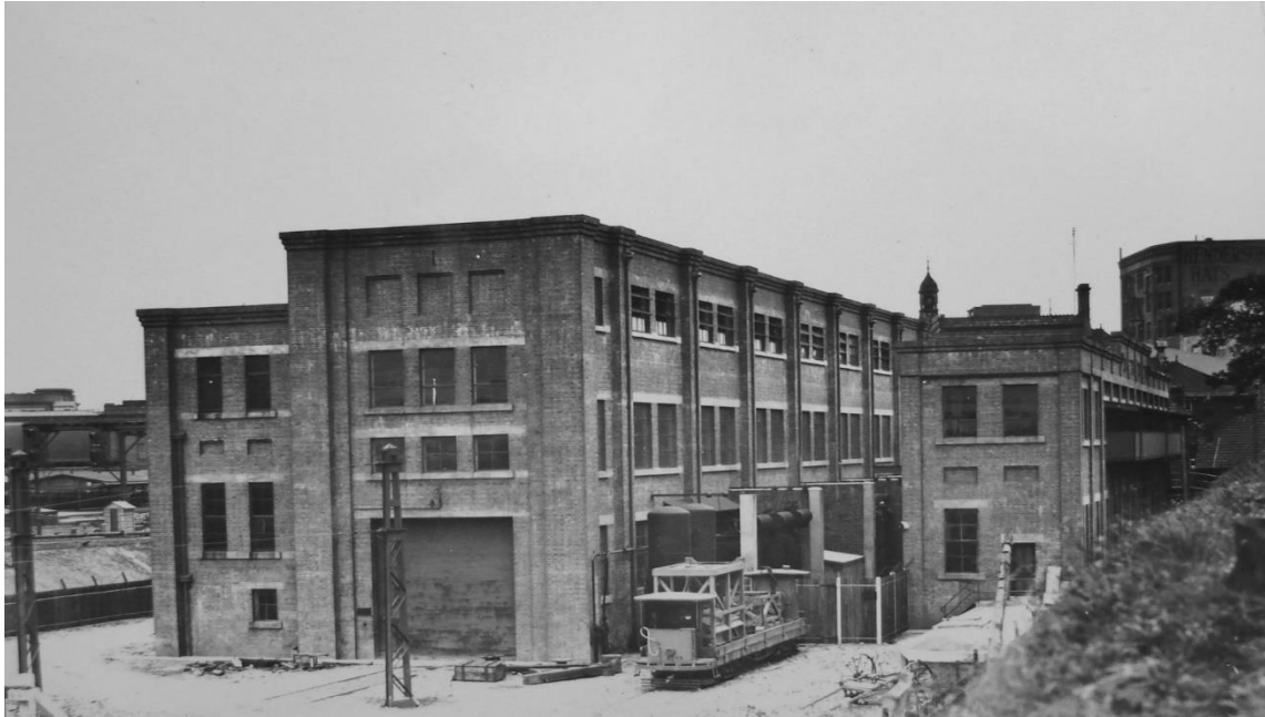
Figure 92: The Prince Alfred Substation c.1928, showing the main substation on the left, switching house to the right and outdoor transformers in the centre. 197
