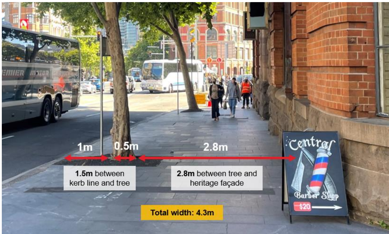
Figure 8: Existing Footpath Measurements (Segment 1: Lee Street Footpath, adjacent Adina Hotel)
