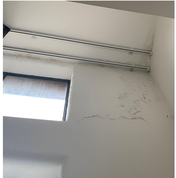
Figure 8 Detail view to minor water damage and mould within Unit 73 (Level 5).
