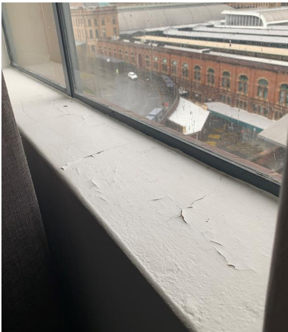
Figure 9 Detail view to minor paint flaking to window interior within Unit 77 (Level 5).
