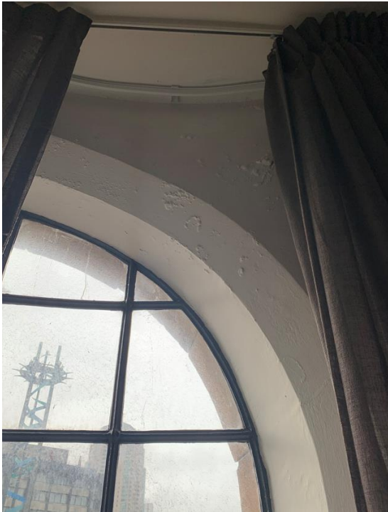
Figure 5 Detail view to minor paint bubbling to window interior within Unit 38 (Level 3).
