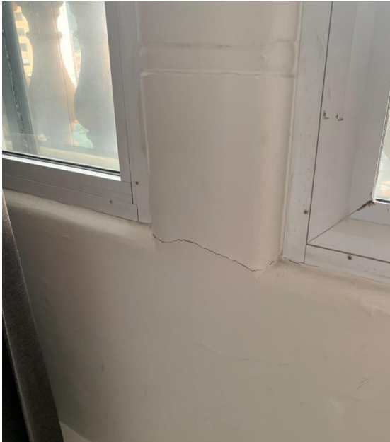
Figure 7 Detail view to minor paint cracking to original fabric wall in Unit 62 (Level 4).
