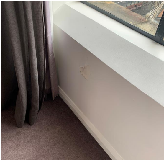
Figure 1 Minor paint peeling noted in Unit 10 (Level 1).
