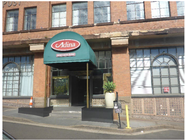
Figure 38 – Awning and accessible entrance of the north elevation. Note the extant stallboard and pavement lights.
