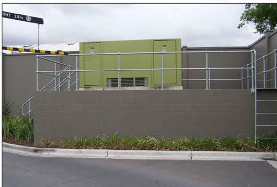
Figure 51 - Example substation raised above 1:100 flood level
