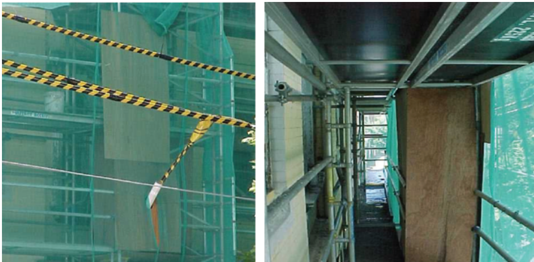
Figure 11 – Enclosure of overhead powerlines
