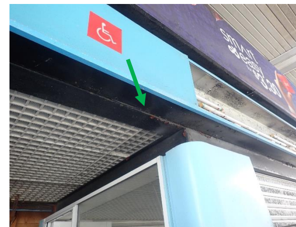
Photo 60: Former Monorail Station – non-lead based black paint to the ticket booth structure
