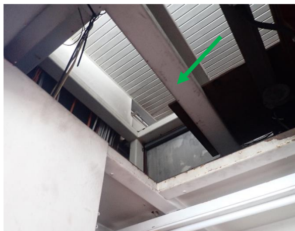
Photo 59: Former Monorail Station – non-lead based grey paint to the steel framework
