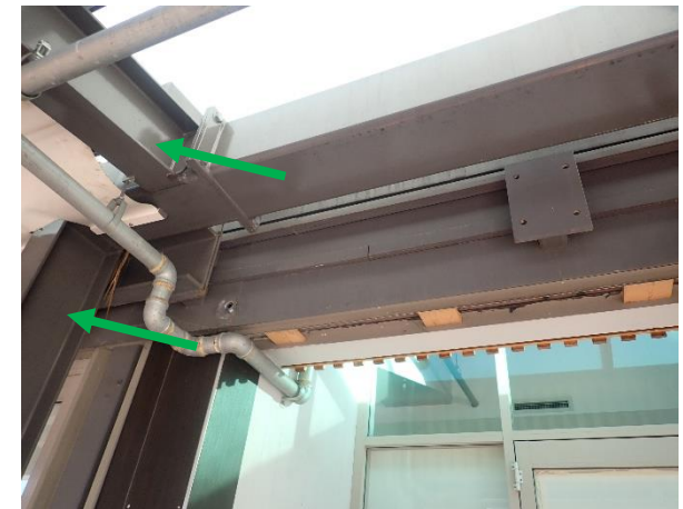
Photo 12: Harbourside – non-lead based grey paint to the external steel framework
