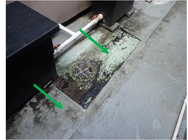
Photo 45: Harbourside – non-asbestos containing upper and lower waterproofing membranes to the cooling tower area on Level 3
