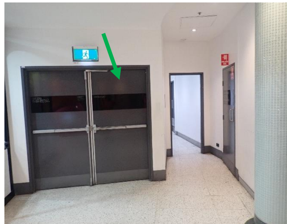
Photo 35: Harbourside – non-lead based grey paint to the common area doors and frames on Level 2
