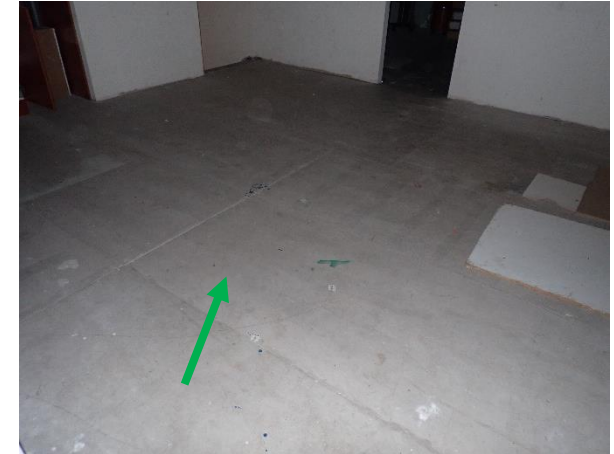
Photo 33: Harbourside – non-asbestos containing compressed fibre cement sheeting to the mezzanine floor of Shop 402 (formerly World Newsagency) on Level 2
