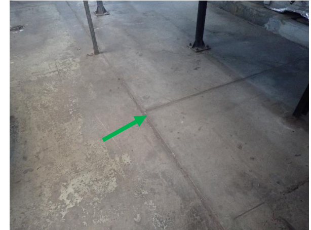
Photo 21: Harbourside – non-asbestos containing bituminous floor expansion joints within the chiller plant room on Level 1
