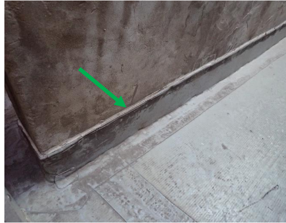
Photo 44: Harbourside – non-asbestos containing white mastic sealant to the edge of the waterproofing membrane throughout the cooling tower area on Level 3
