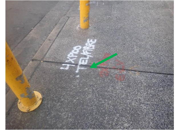
Photo 9: Harbourside – non-asbestos containing bituminous floor external expansion joints
