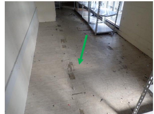
Photo 30: Harbourside – non-asbestos containing cream vinyl flooring to the rear store rooms of Shop 419 (formerly Glue) on Level 2
