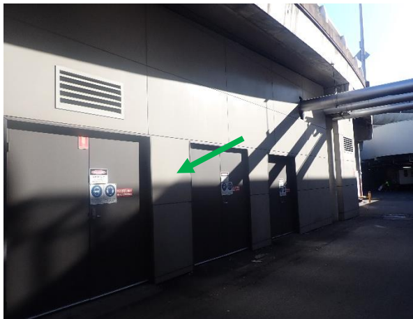
Photo 10: Harbourside – non-asbestos containing compressed fibre cement sheeting to the chiller plant room/Ausgrid Substation external cladding
