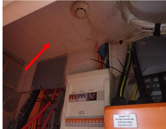
Photo 38: Harbourside – assumed SMF insulation to floor, wall and ceiling penetrations on Level 2
