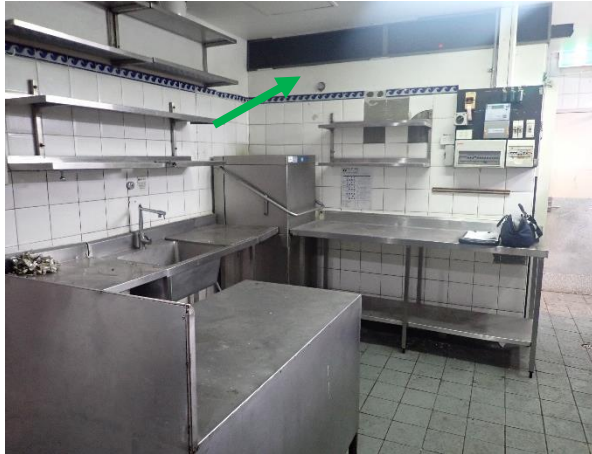
Photo 19: Harbourside – non-asbestos containing fibre cement sheeting to the kitchen/back of house wall linings in Shop 293 (formerly Toro) on Level 1
