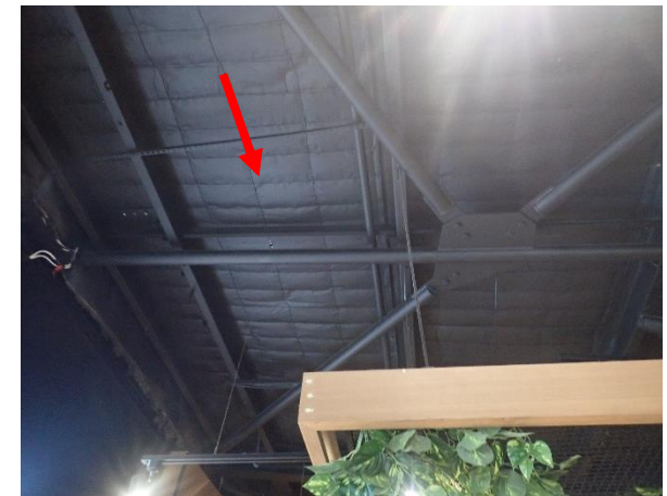
Photo 36: Harbourside – assumed SMF insulation to the roof sarking within the ceiling cavities/plant rooms on Level 2
