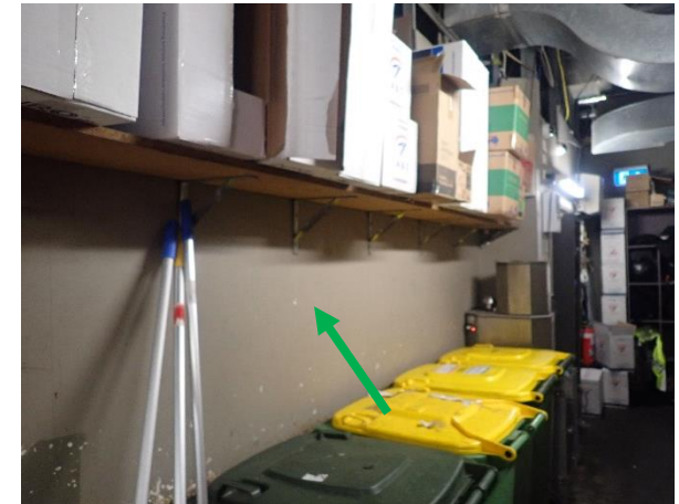
Photo 18: Harbourside – non-asbestos containing fibre cement sheeting to the back of house/kitchen wall linings in Shop 198 (The Watershed) on Level 1
