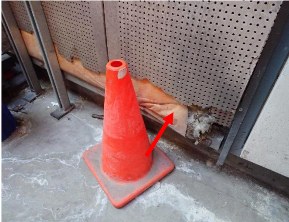
Photo 49: Harbourside – assumed SMF insulation to the walls of the cooling tower area on Level 3
