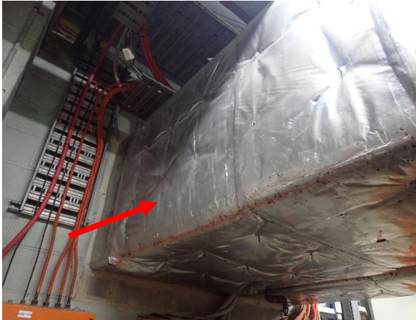
Photo 25: Harbourside – assumed SMF insulation to the HVAC ducting throughout the ceiling cavities/plant rooms on Level 1
