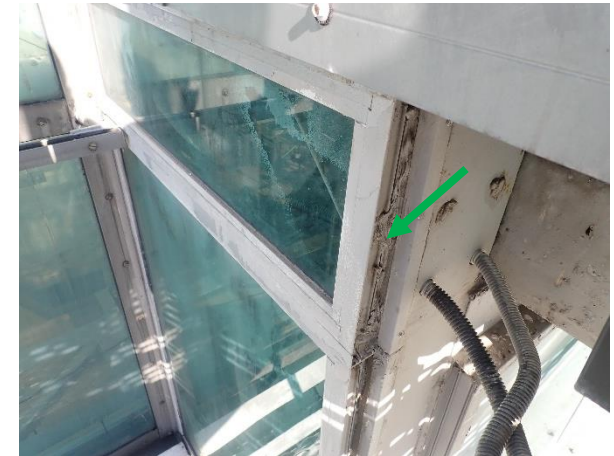
Photo 3: Harbourside – non-asbestos containing grey mastic sealant to the external steel framework
