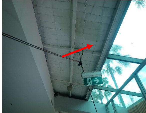
Photo 26: Harbourside – assumed SMF insulation to the roof sarking within the ceiling cavities/plant rooms on Level 1
