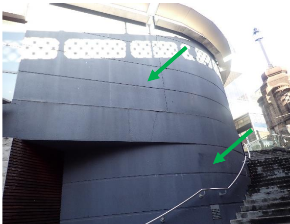
Photo 4: Harbourside – non-asbestos containing compressed fibre cement sheeting to the external cladding
