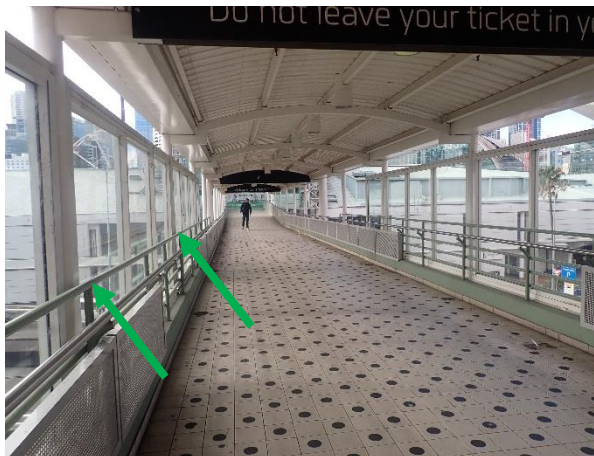
Photo 55: Pedestrian Link Bridge – non-lead based green paint to the handrails and balustrades
