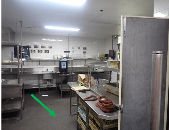
Photo 31: Harbourside – non-asbestos containing black membrane to the kitchen floor of Shop 321/357 (formerly Hard Rock Café) on Level 2
