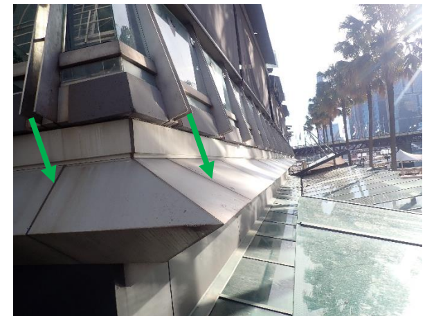
Photo 6: Harbourside – non-asbestos containing mastic sealant to the external metal cladding
