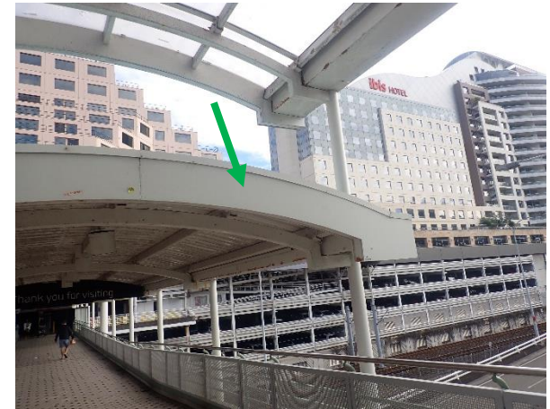
Photo 54: Pedestrian Link Bridge – non-asbestos containing compressed fibre cement sheeting to the east and west fascia cladding
