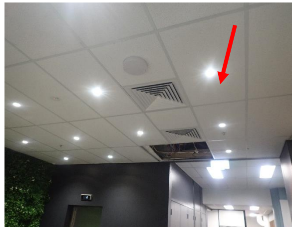
Photo 29: Harbourside – assumed SMF suspended ceiling tiles throughout the Mirvac Offices on Level 1
