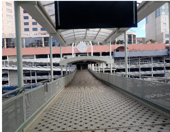
Photo 53: Overview of Pedestrian Link Bridge
