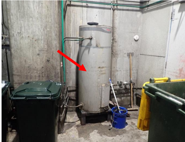
Photo 13: Harbourside – assumed SMF internal insulation to hot water systems within the loading dock
