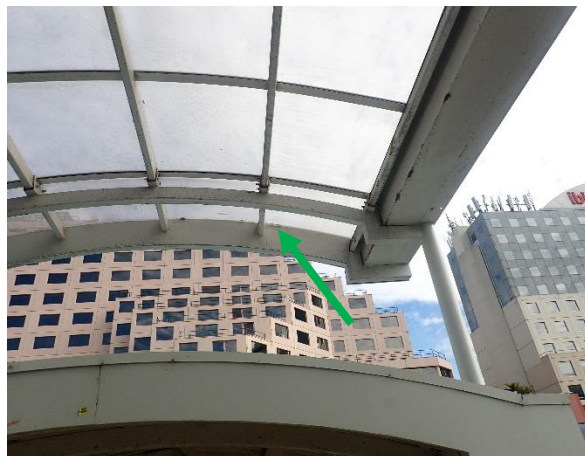
Photo 56: Pedestrian Link Bridge – non-lead based white paint to the steel framework
