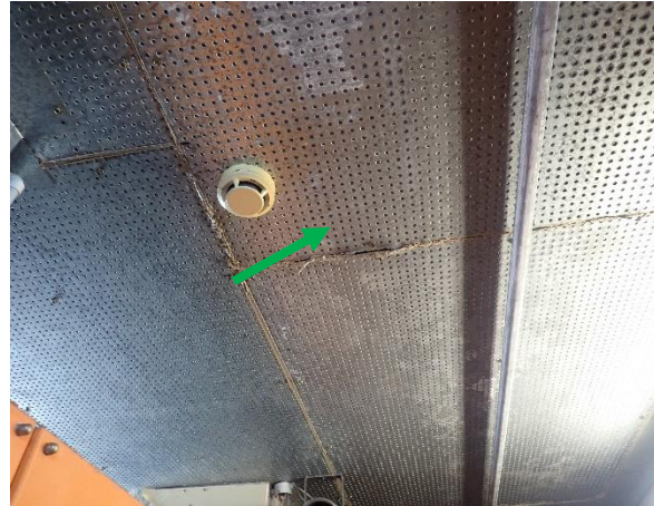
Photo 20: Harbourside – non-asbestos containing fibre cement sheeting to the internal core of the ceiling panels in the main switchroom on Level 1
