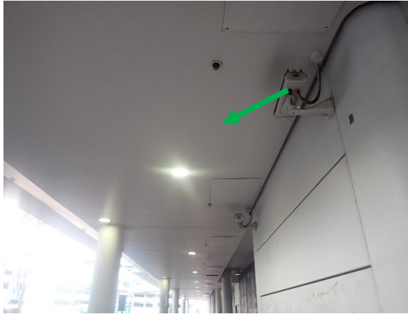
Photo 7: Harbourside – non-asbestos containing fibre cement sheeting to the external soffit linings
