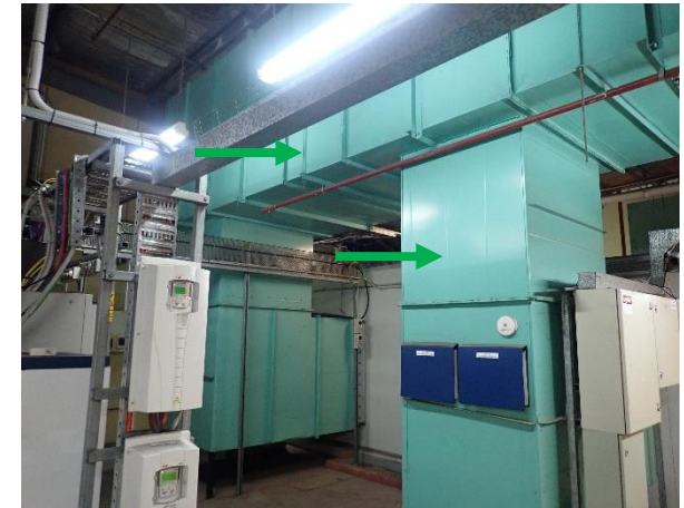
Photo 48: Harbourside – non-lead based aqua paint to the HVAC ducting in the plant room on Level 3
