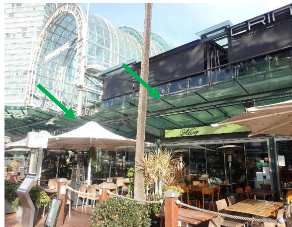
Photo 5: Harbourside – non-asbestos containing black mastic sealant to the glass panel awnings
