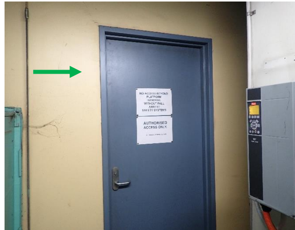
Photo 47: Harbourside – non-lead based cream paint to the plant room walls on Level 3
