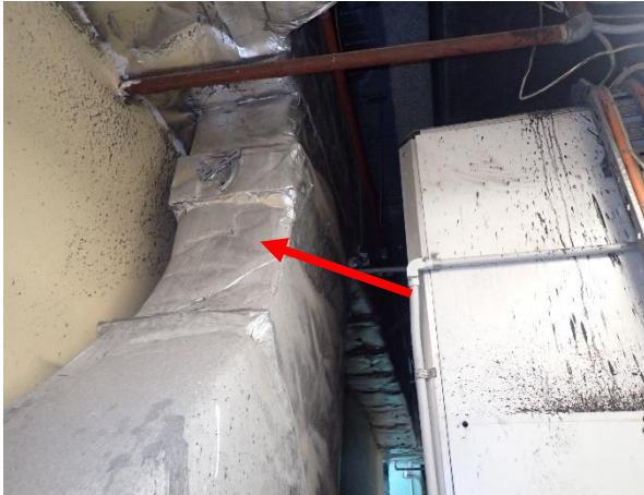
Photo 37: Harbourside – assumed SMF insulation to the HVAC ducting within the plant room on Level 2
