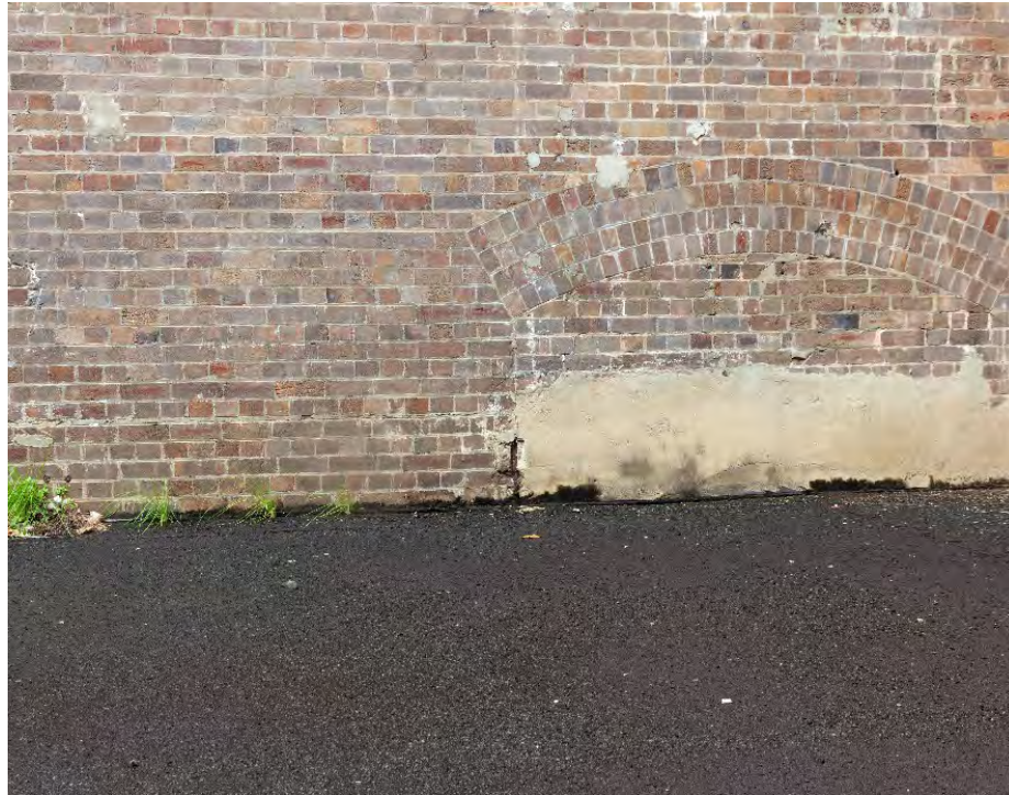
Pump House Viewpoint 9: Original brick archway obscured by construction of modern Level 1 surface
