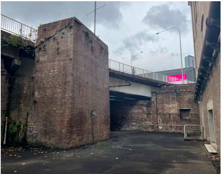
Pump House Viewpoint 5: Level 1, William Henry Street bridge resting on remnant north and eastern pump house walls, remnant chimney section.
