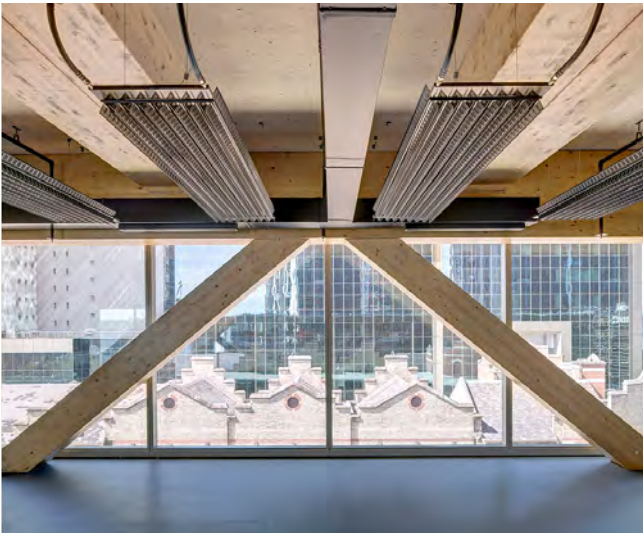
Daramu House CLT Structure, Tzannes Image credit: Brett Boardman
