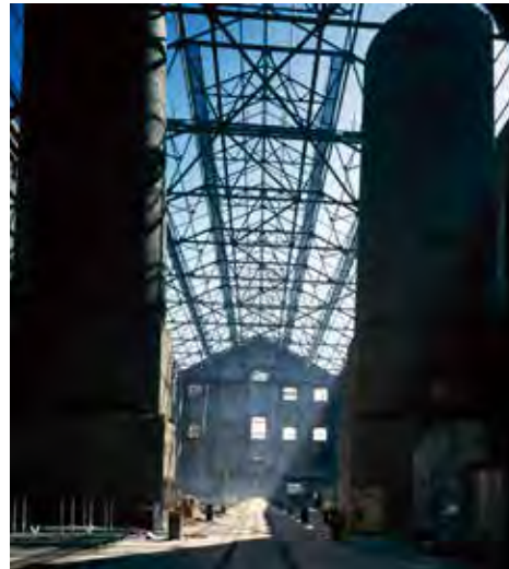
11 | Boiler Hall during construction. The 1902 chimneys are now used as part of the air conditioning system.
