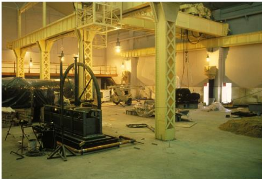
The original Engine House of Ultimo Power House (UPH) with the later Turbine House in the foreground. The gantry cranes are original to the Ultimo Power House and there are 3 in total in situ. Two were made in USA in 1899 and one in Australia in 1929.
