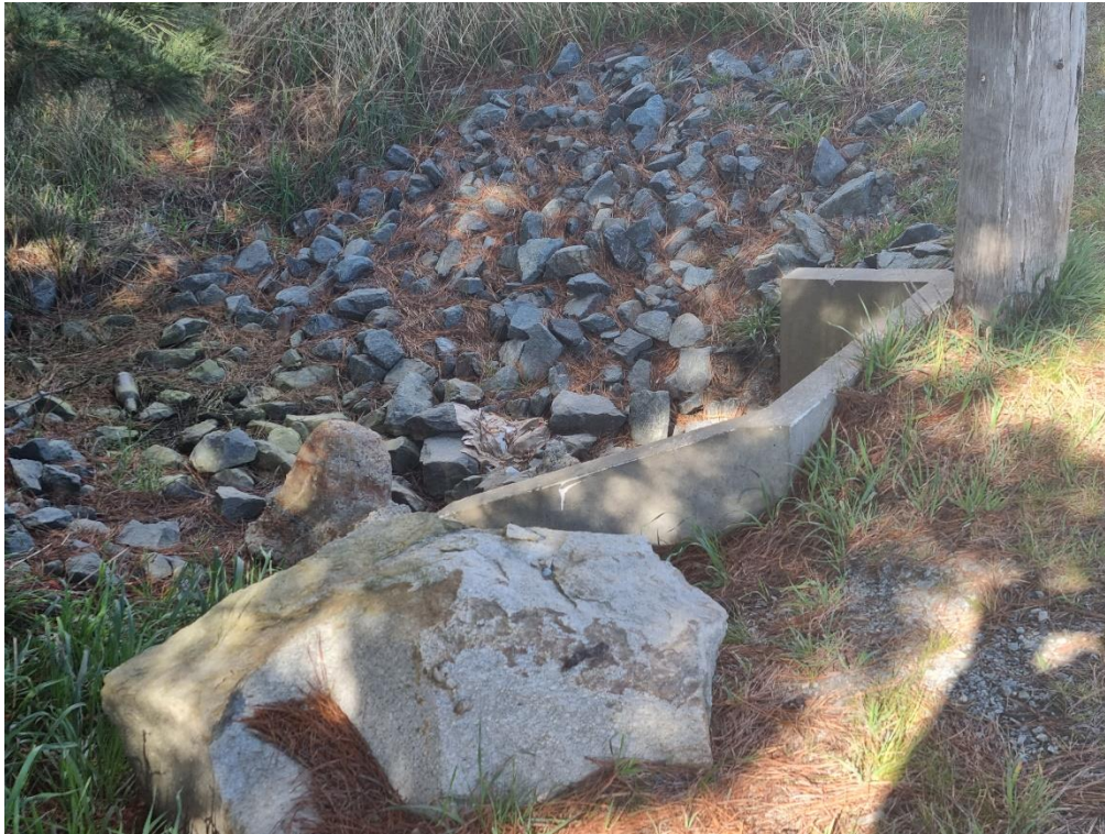
FIGURE 4 CULVERT ACROSS THE INTERSECTION (NORTH HEADWALL AND SWALE SHOWN)
