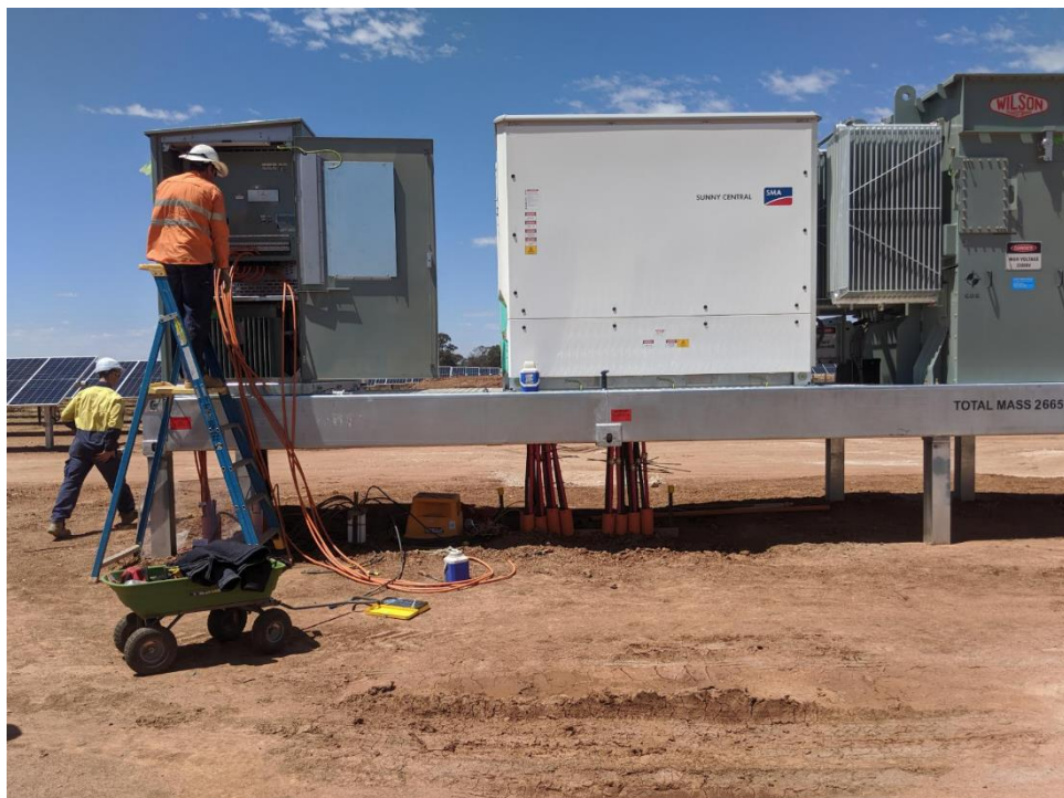
Figure 1-8 PCU installed on pile foundation (Courtesy of Octopus Investments Australia)
