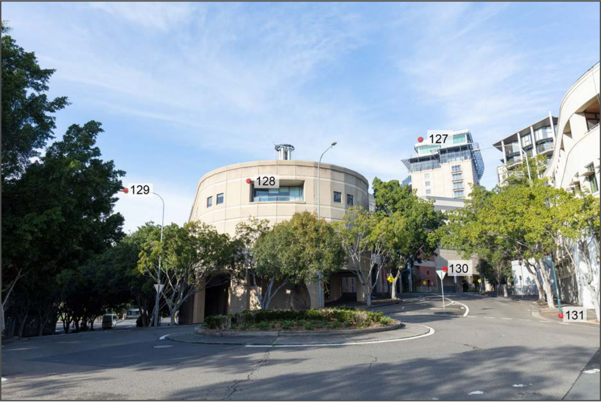
ORIGINAL PHOTOGRAPH INCLUDING SURVEYED ALIGNMENT DATA
