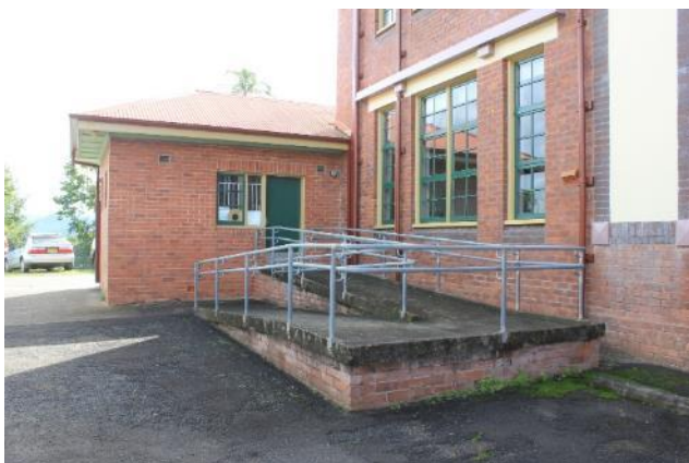
Plate 7.3 Disabled access ramp to extension. Source: EMM 2021.
