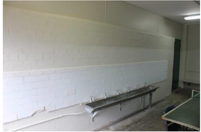
Plate 5.15 Ground Level – Storage partition wall. Source: EMM 2021.
