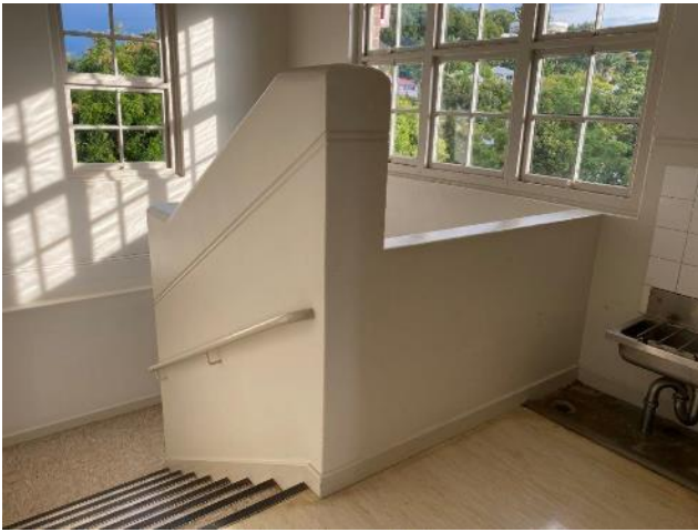
Plate 5.26 Level 2 – western circulation stairwell. Source: EMM 2021.
