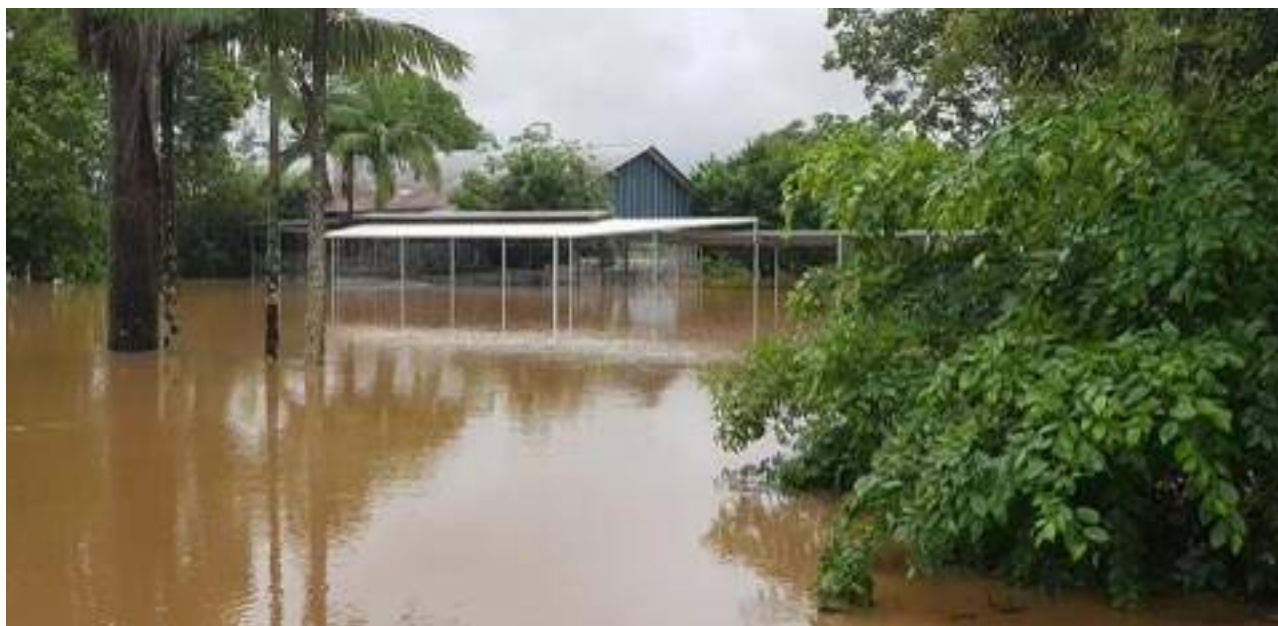
MEPS site and buildings flood impacted
