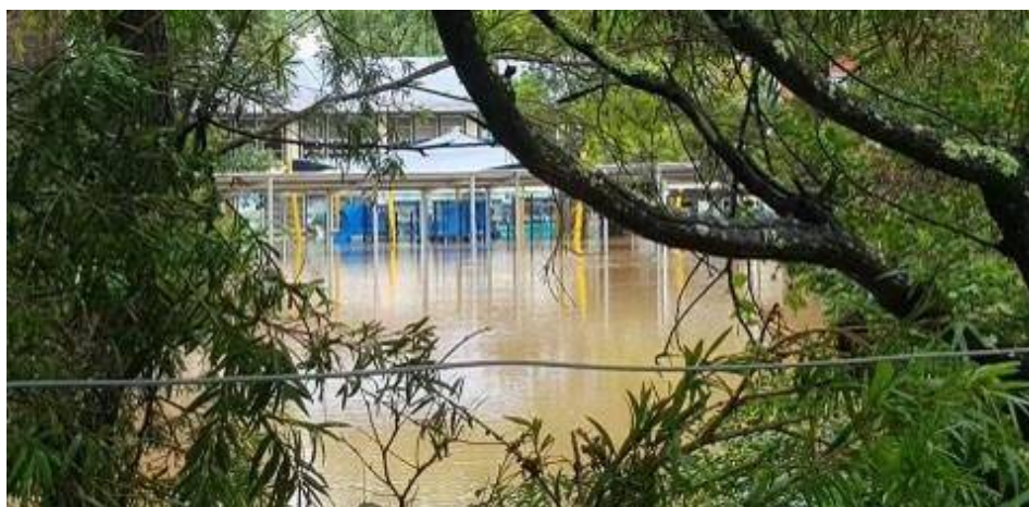
MEPS building flood impacted
