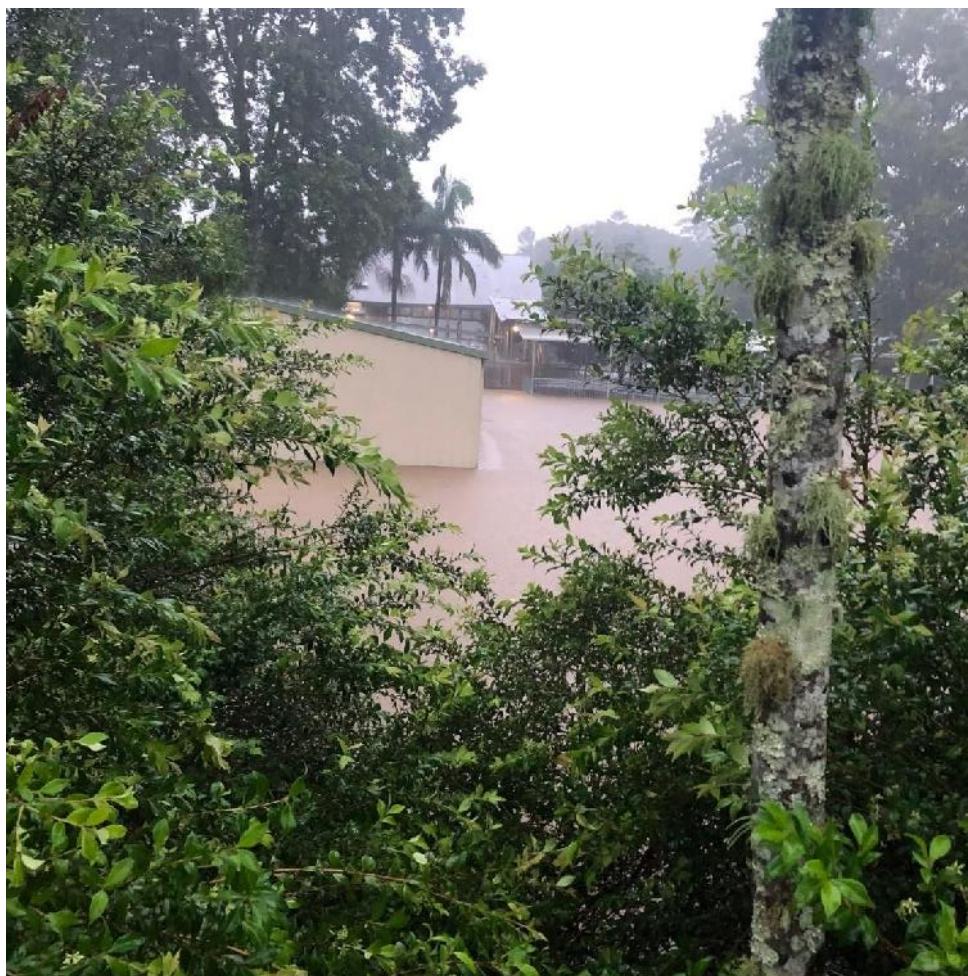
MEPS site and buildings flood impacted
