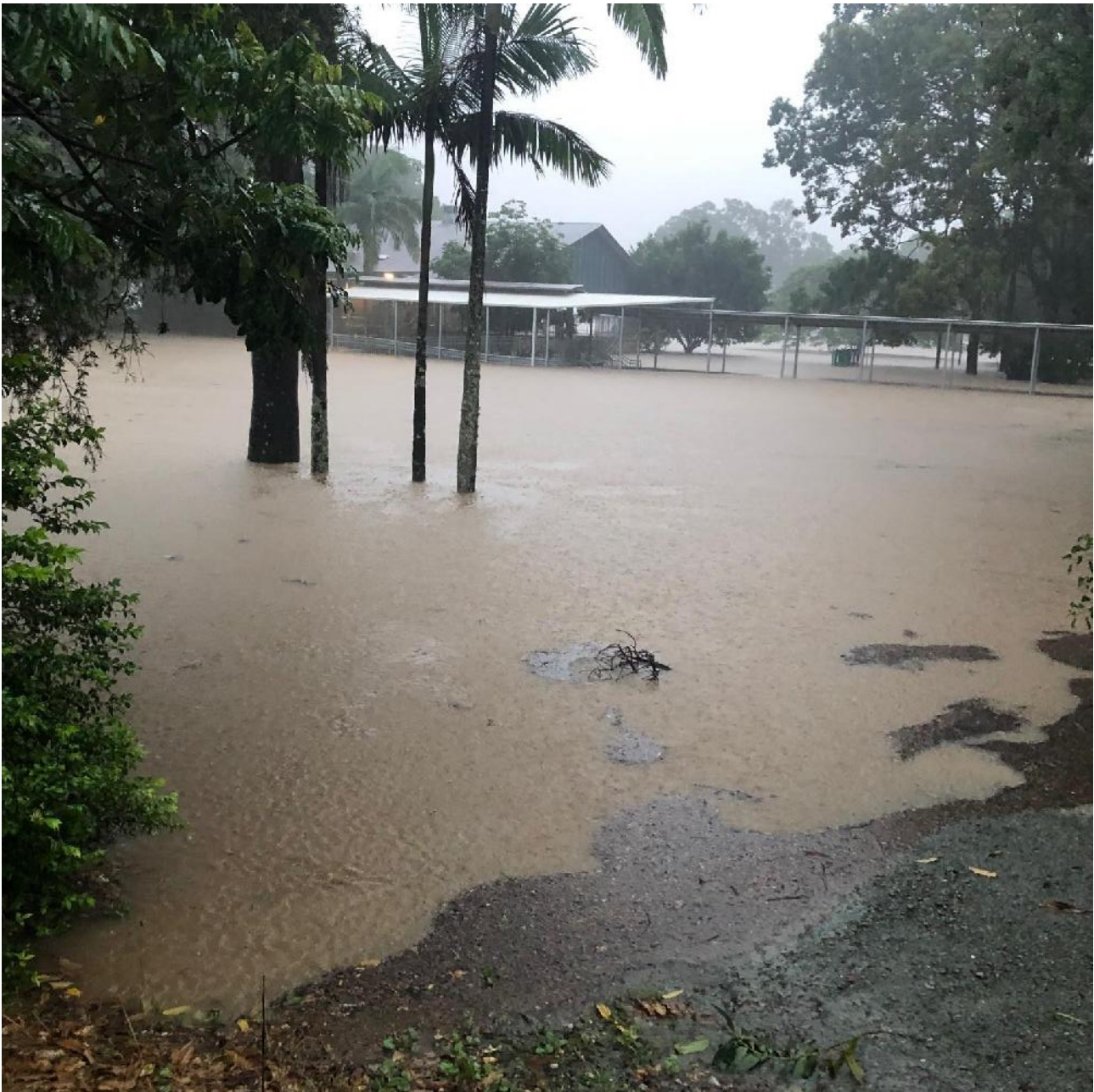
MEPS site and buildings flood impacted
