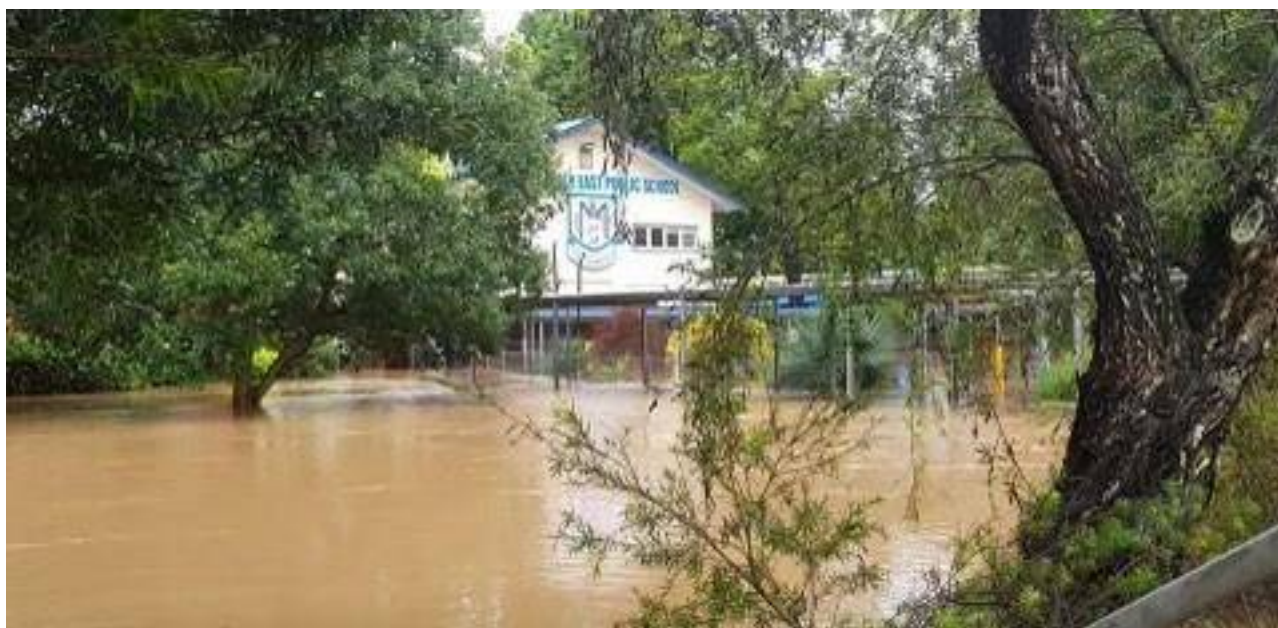
MEPS site and buildings flood impacted
