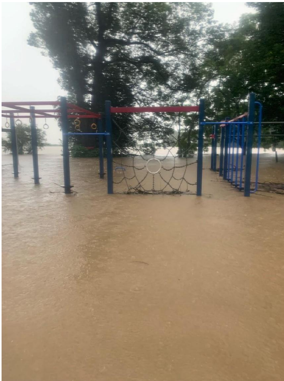
MEPS playground flood impacted
