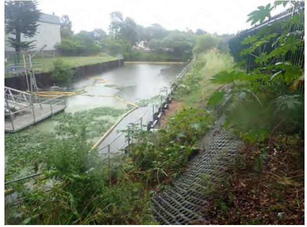
Figure 13 – View north-west of embankment above retention basin
