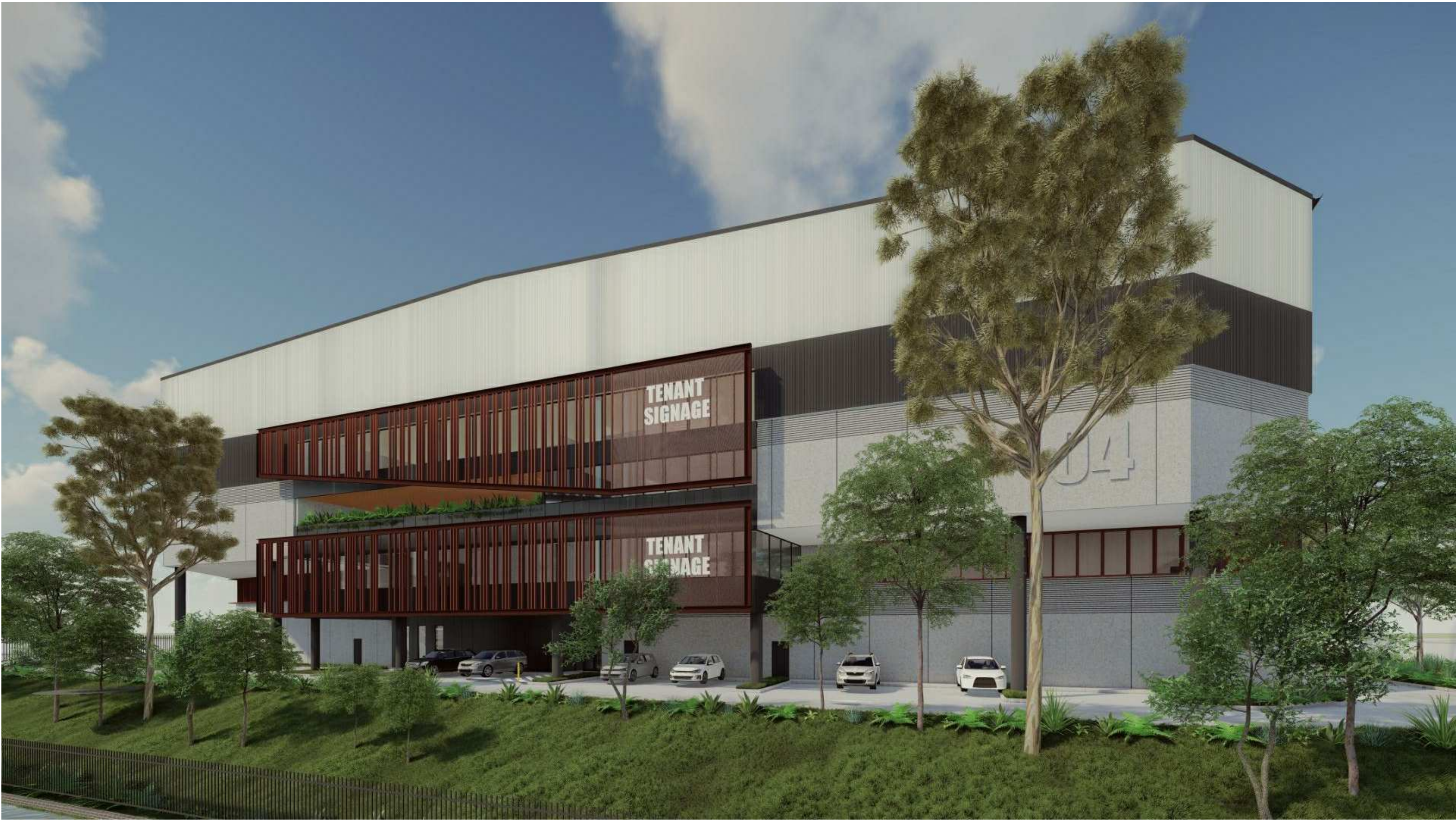
OFFICE 2 & 4 STREET VIEW FROM SOUTH
