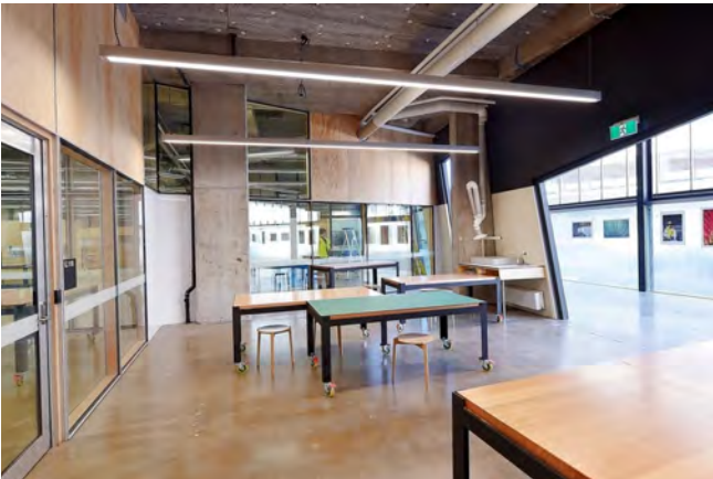
Exposed services for central spaces for industrial feel, hidden services in offices
