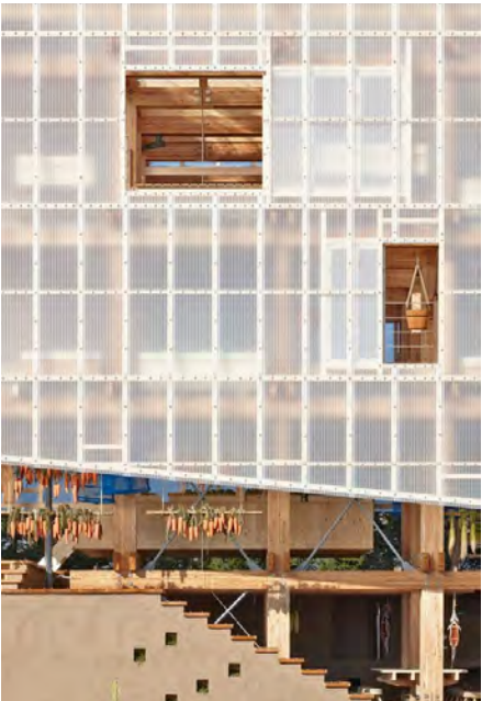
Polycarbonate sheets as a skin, for diffused lighting in warehouse spaces
