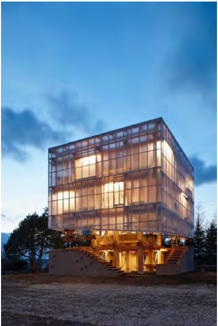
Polycarbonate sheets as a skin, for diffused lighting in warehouse spaces
