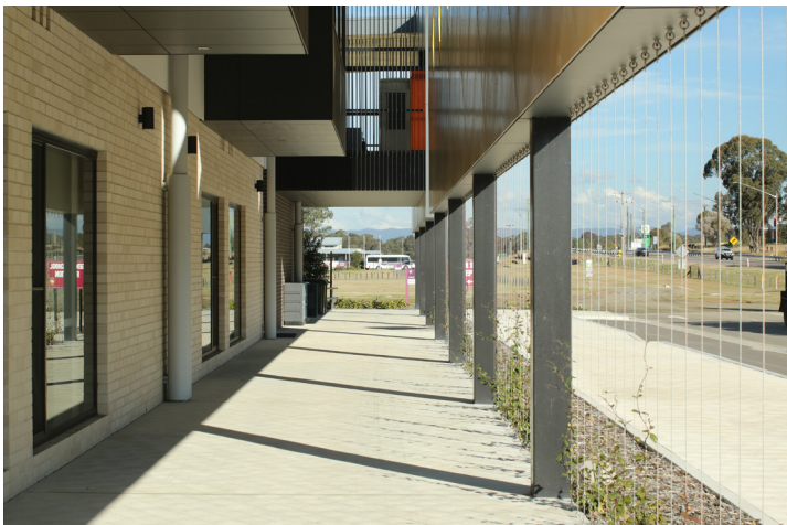
7. Covered walkway along new building
