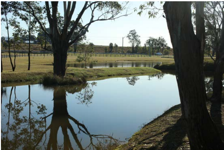
13. View across dam toward bund wall
