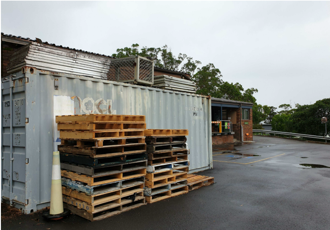
View 3 provides a closer view of the nutrition building.
