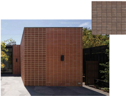
01 STACKED BOND BRICKWORK
