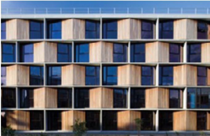
Figure 1 - Out of phase facade
