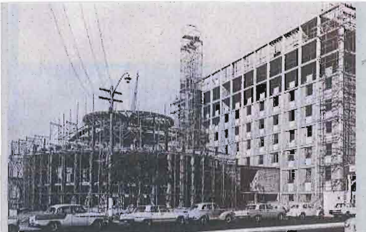
Figure 41 The site during construction works (International House, A decade of Achievement , 1977)
