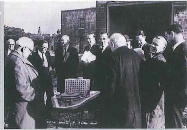
Figure 39 The first inspections to the construction site with the architect. (Fischer, op.cit. , p. 107)
