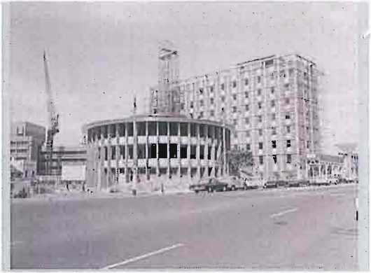
Figure 46 The site during construction works (NAA, http://recordsearch.naa.gov.au/scripts/PhotoSearchItemDetail.asp?M=0&B=7555519 , 1966)
