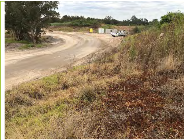
Photo 11. Weed growth on bund west of plant
