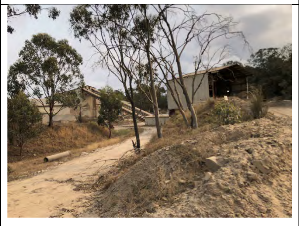
Photo 6. PCT 849 location shot with crusher in background
