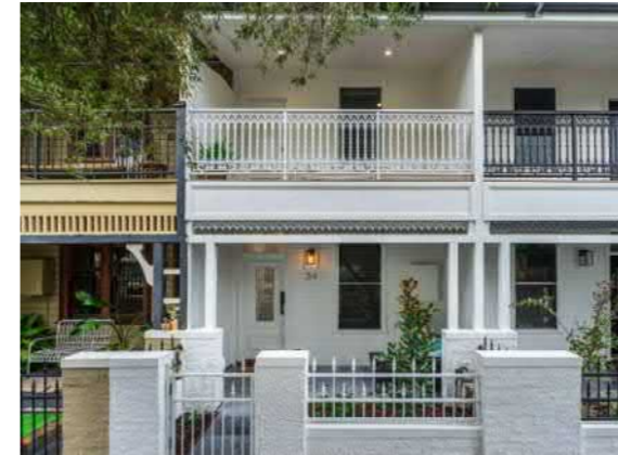
Recently renovated weatherboard terraces
