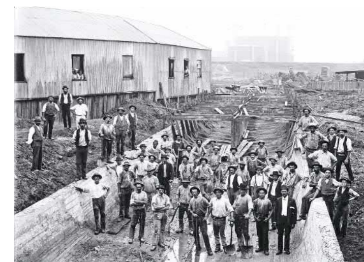
Construction of Cottage Creek Stormwater Drain, image courtesy of Hunter Living Histories
