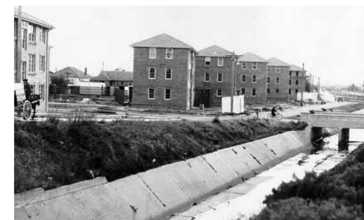
Stormwater Drain on Parkway Avenue Adjacent to Park Site, image courtesy of Hunter Living Histories
