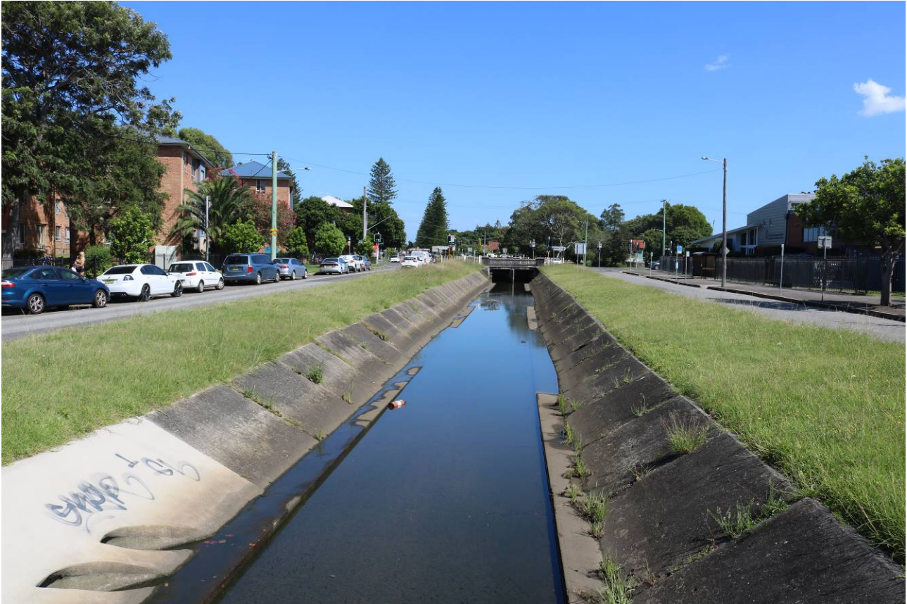
Photograph 4 – Parkway Avenue along site frontage.
