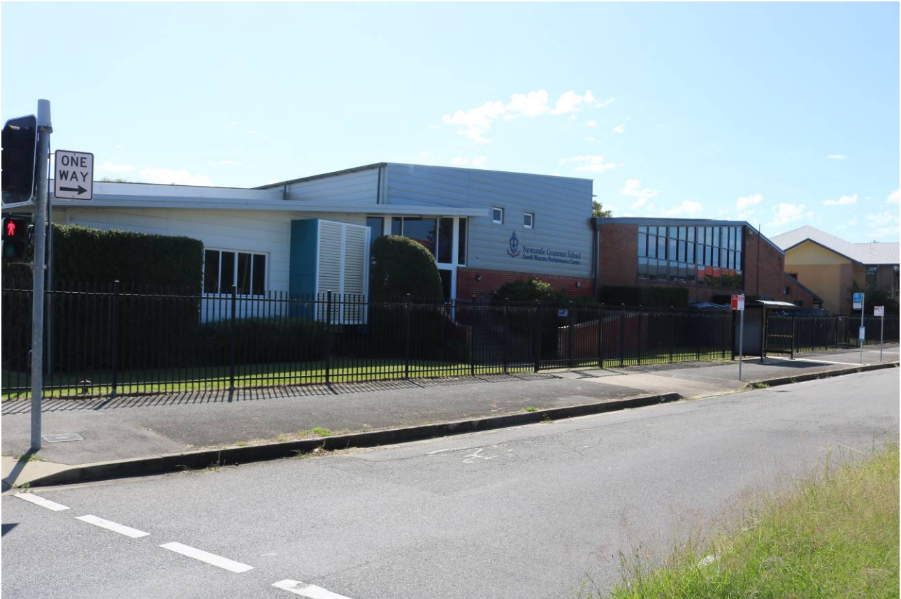
Photograph 1 – Development site from Parkway Avenue
