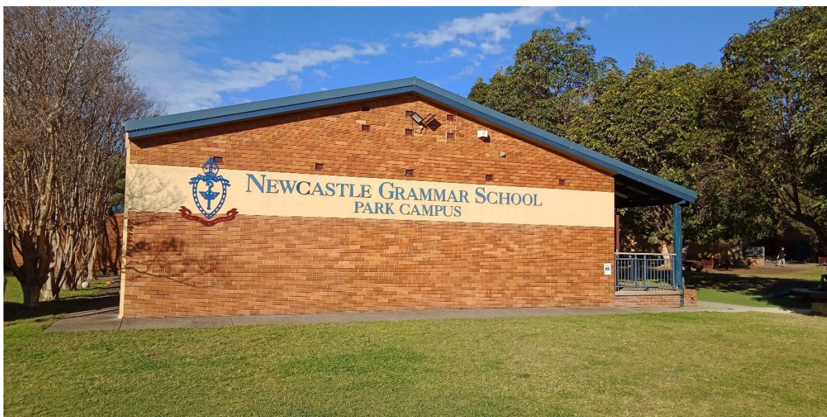
Plate 2 Single storey building at rear
