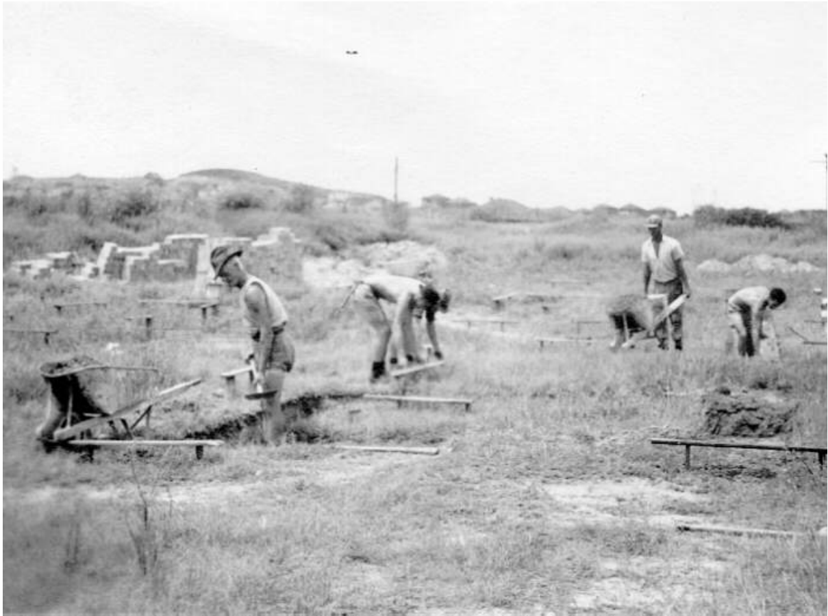
Figure 5 Workers preparing land for the flats at Parkway Avenue 1950
