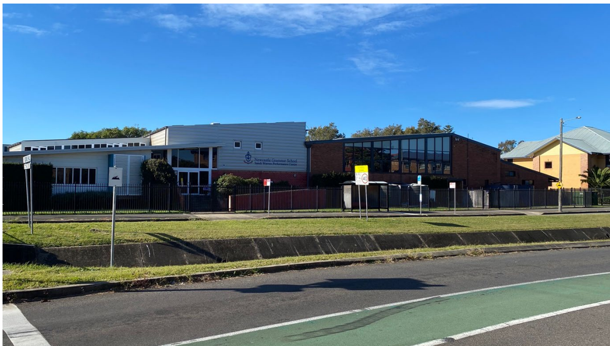
Plate 1 View northwest of the Parkway Avenue frontage of Newcastle Grammar School.
