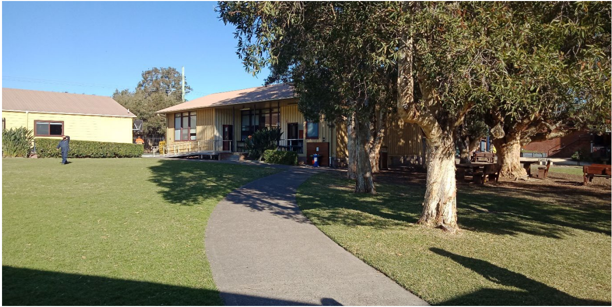
Plate 3 Single storey buildings at rear
