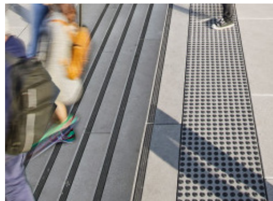
SF1 - CONCRETE STAIRS
