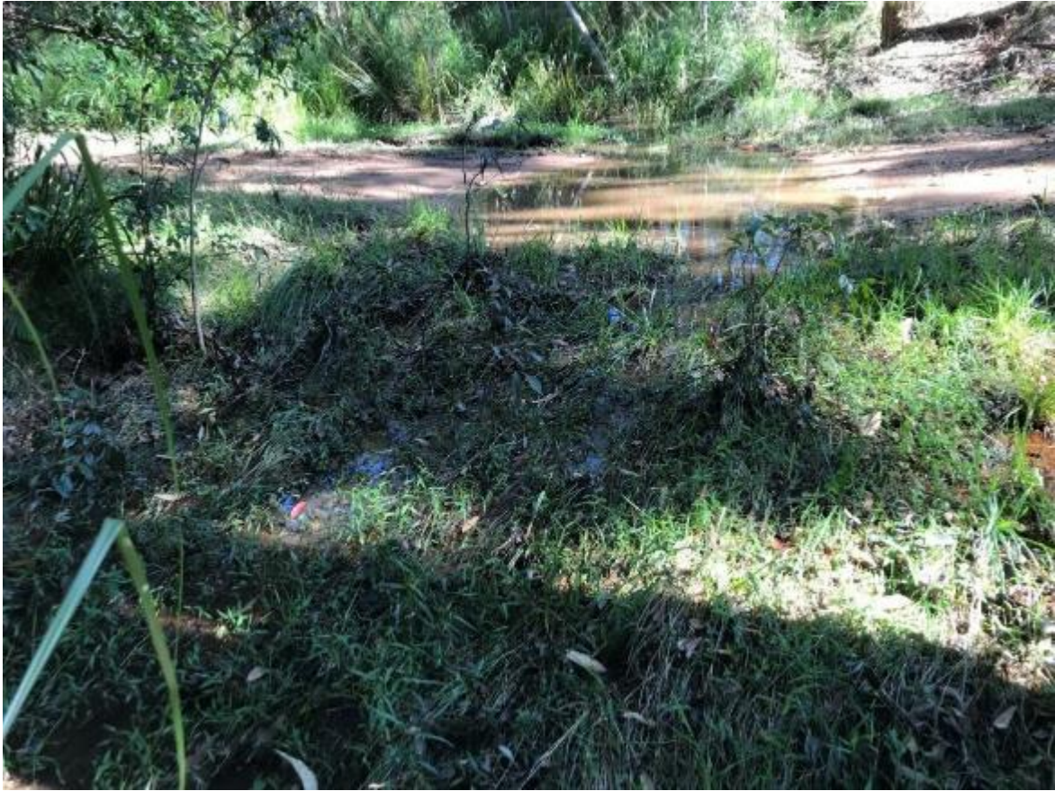
Plate 4: Looking upstream at ST2 Deep Creek Rd crossing.
