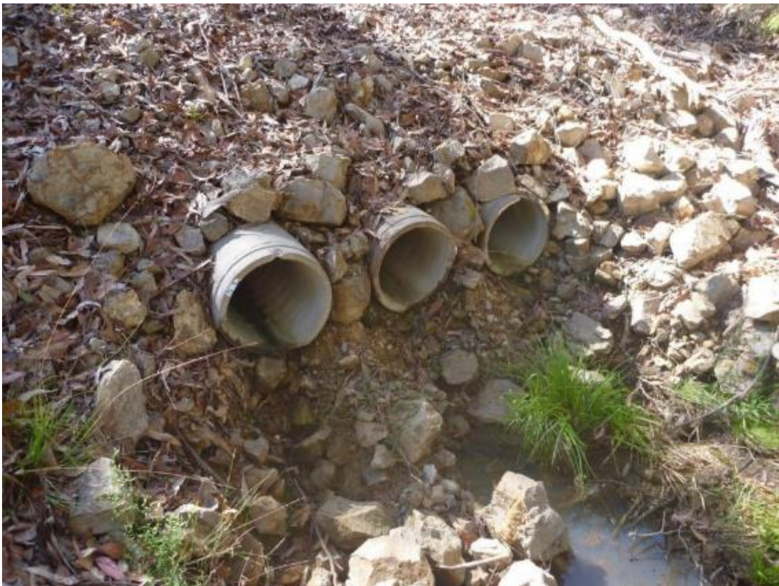
Plate 38: NT6 pipe culverts on the downstream side of the constructed track.
