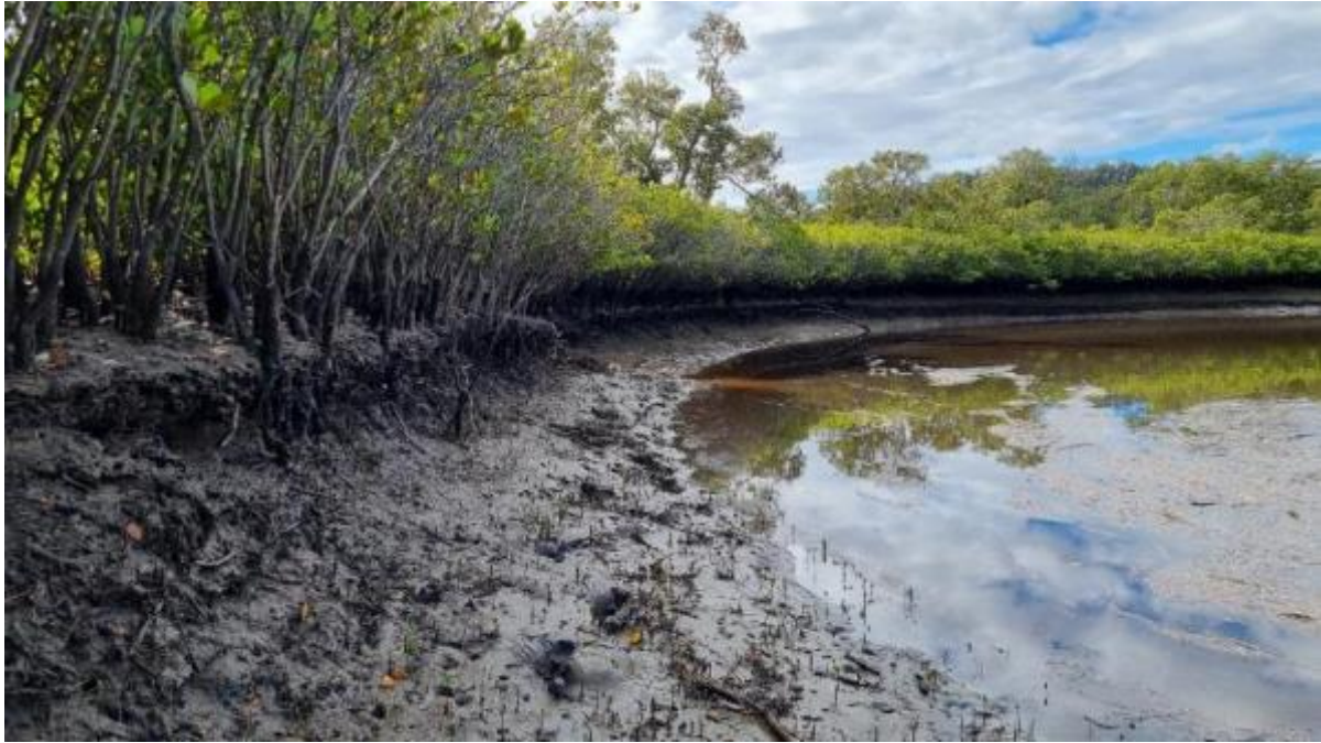
Figure 18 Looking downstream along incised and undercut banks at DCDn.
