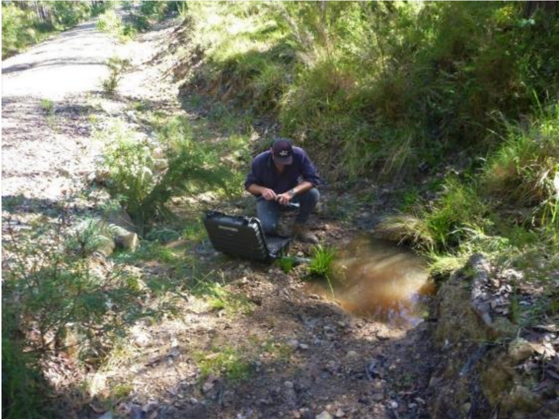
Plate 37: Looking west along the constructed track crossing over NT6, showing the small surface pool on the upstream side of the pipe culverts.
