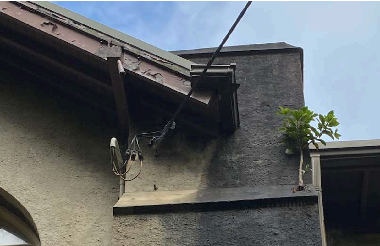
Photo. 10. Vegetation growing on the masonry is to be removed and the cracks repaired.
