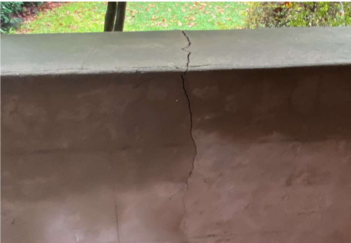
Photo. 12. Cracks in masonry are to be repaired with minimal disturbance to original heritage fabric.
