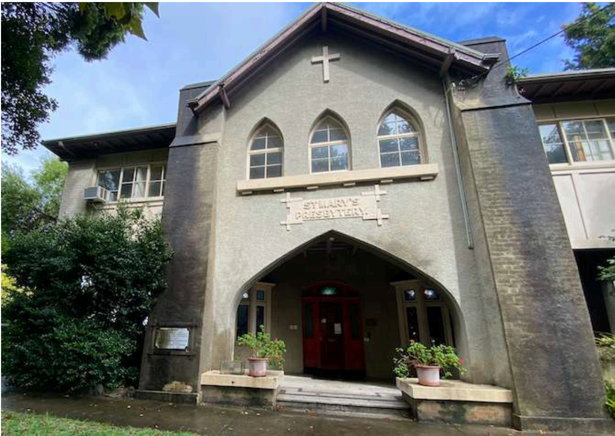
Photo. 7. All of the external brickwork and masonry is to be professionally cleaned by an experienced contractor with a proven record of satisfactory work on heritage buildings.
