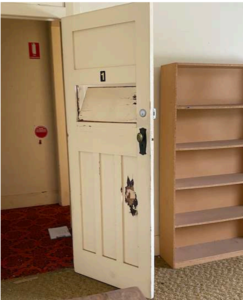
Photo. 39. The damaged heritage door on the first floor at the rear of the Presbytery is to be replaced with a matching heritage door. Preferably a heritage door sourced from a heritage building supply centre.
