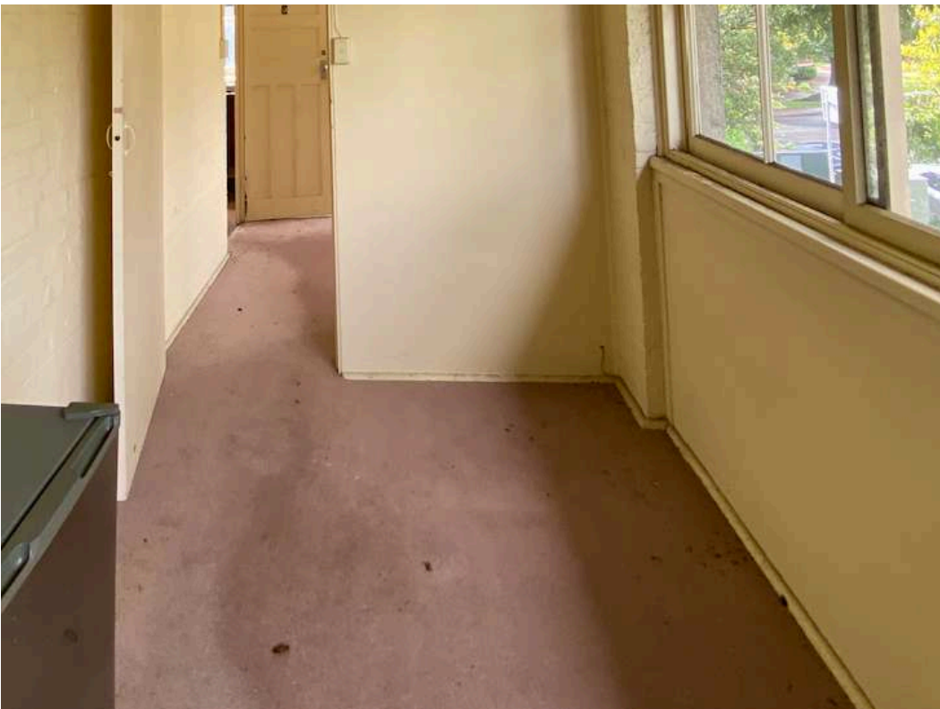
Photo. 14. Prior to the removal of the existing windows to reinstate the first floor verandahs on the northern and southern elevations (demolition) both internal and external cladding is to be examined to ensure the cladding material is not asbestos sheet.
