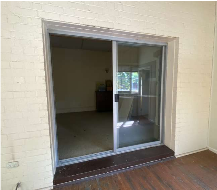
Photo. 28. The Aluminium sliding door at the north end of the eastern elevation on the first floor is to be removed. Details of the proposed new timber door or window are to be approved by the nominated heritage consultant.
