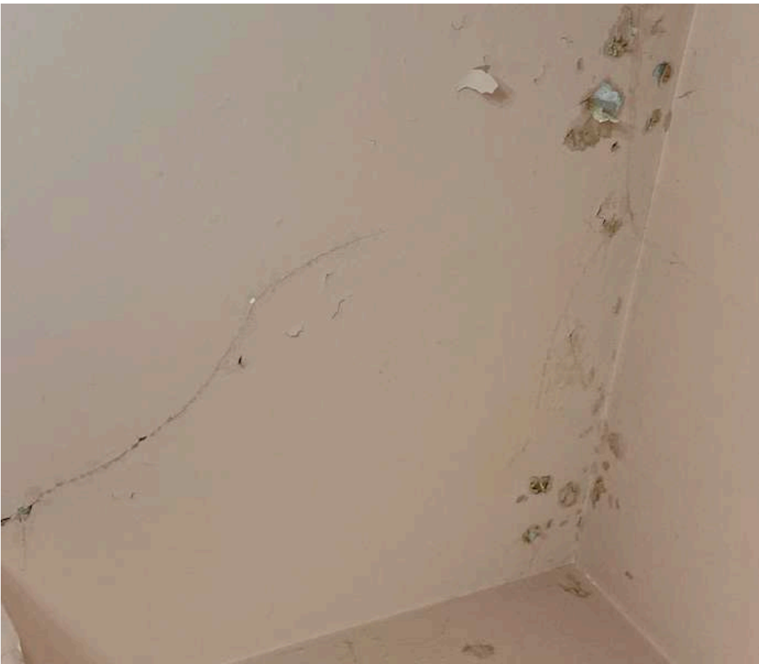
Photo. 37. The water damaged ceiling in the ground floor room on the southern side is to be repaired and the hand basin in the room directly above investigated for water leaks.
