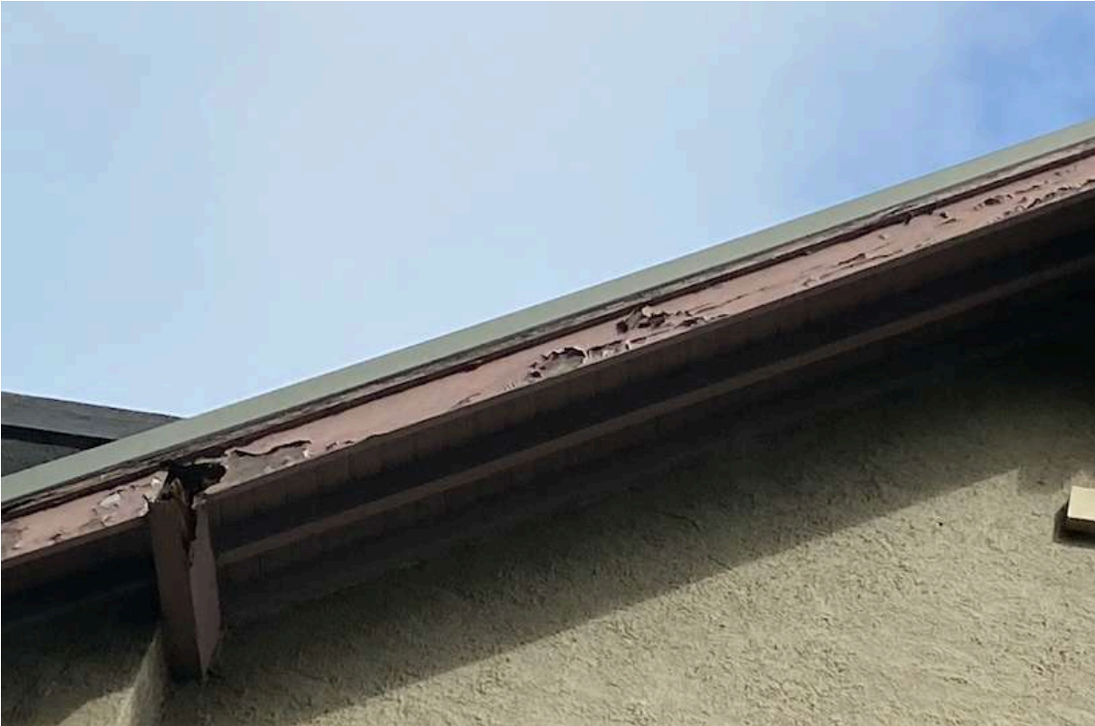
Photo. 5. All barge boards, fascia and eaves lining boards are to be inspected for damage and repaired where required by an experienced contractor with a proven record of satisfactory work on heritage buildings prior to properly preparing and repainting.
