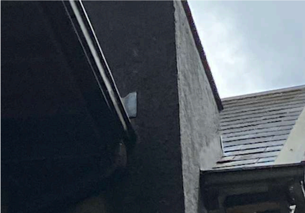
Photo. 3. The slate roof appears to be in a serviceable condition. The roof slate and all associated flashings are to be inspected by a heritage roof slate contractor.
