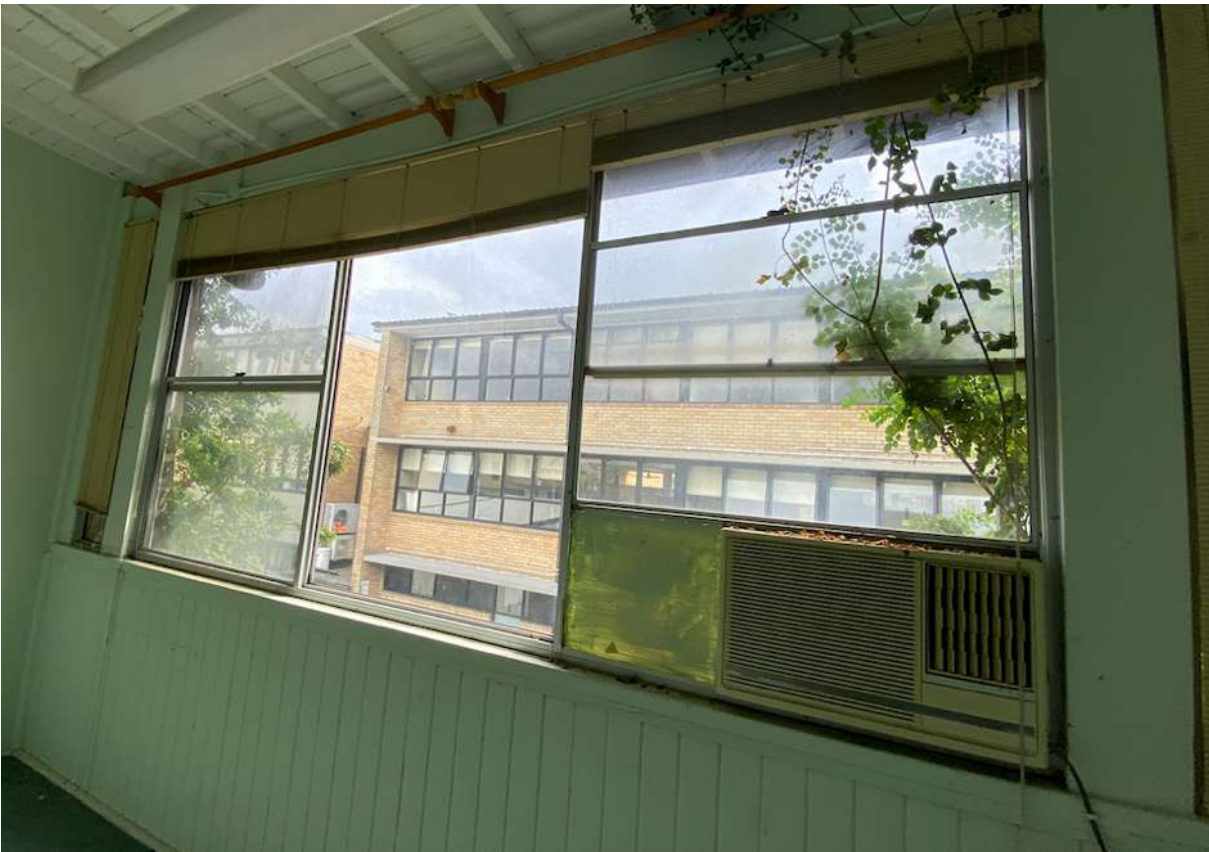
Photo. 17. All aluminium windows and air-conditioning units are to be removed.
