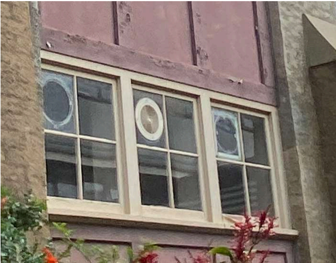
Photo. 22. The ground floor timber windows at the rear of the building on the northern elevation are to be retained or replaced with a sliding timber windows recycled from the first floor verandah.
