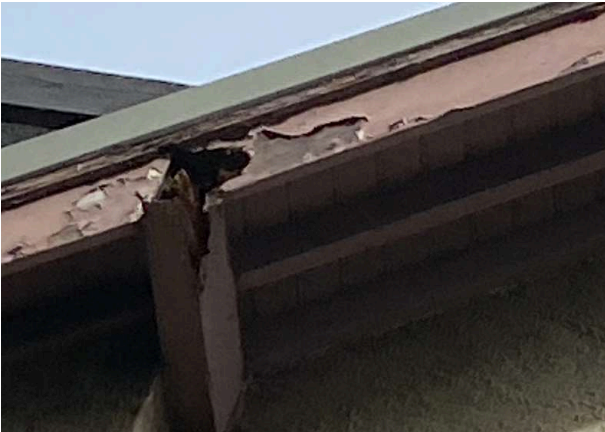
Photo. 6. The rot damaged timber supporting the exposed rafters at the front (east elevation) of the Presbytery is to be repaired.
