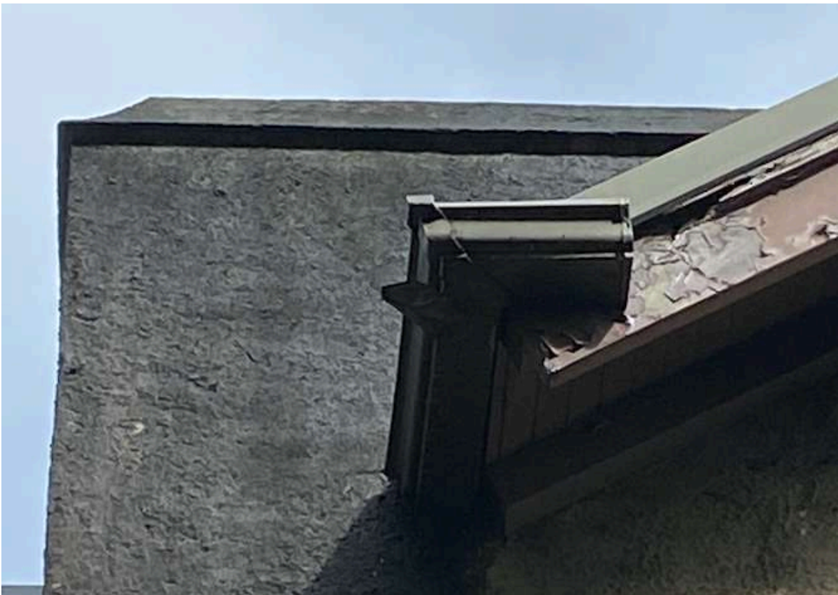
Photo. 4. The gutters and down-pipes are inappropriate and are to be replaced with a copper gutter system.
