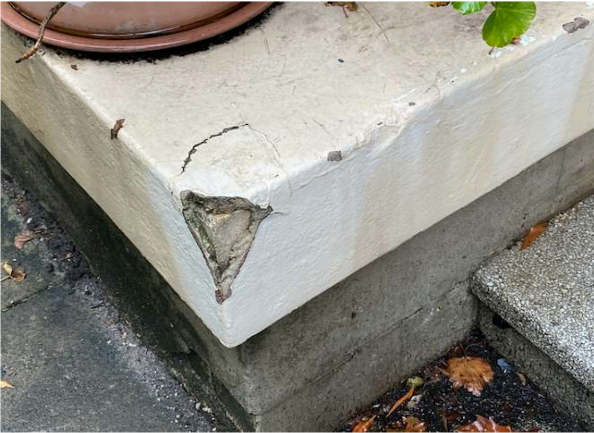
Photo. 9. Damaged render is to be repaired by an experienced contractor with a proven record of satisfactory render repairs.
