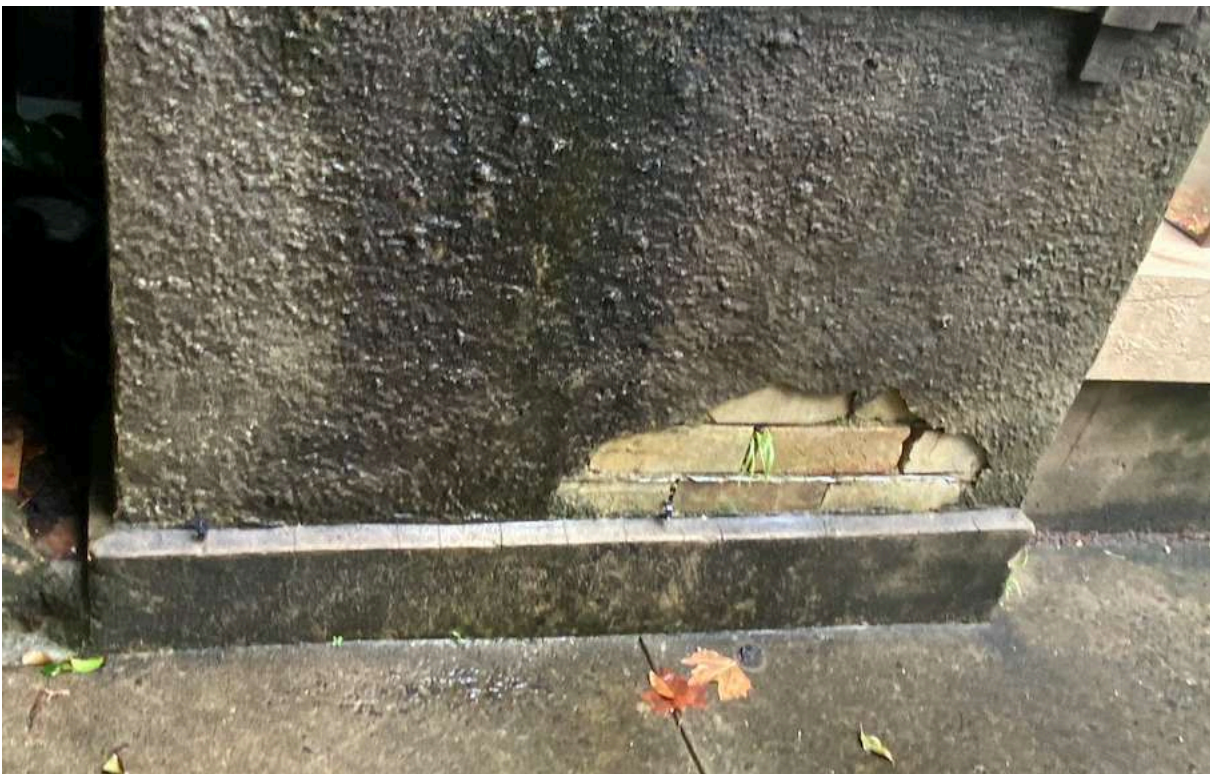
Photo. 8. Damaged tyrolean render is to be repaired by an experienced contractor with a proven record of satisfactory tyrolean render repairs.
