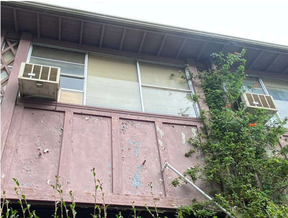
Photo. 15. Prior to the removal of the existing windows to reinstate the first floor verandahs on the northern, east and southern elevations (demolition) both internal and external cladding is to be examined to ensure the cladding material is not asbestos sheet.
