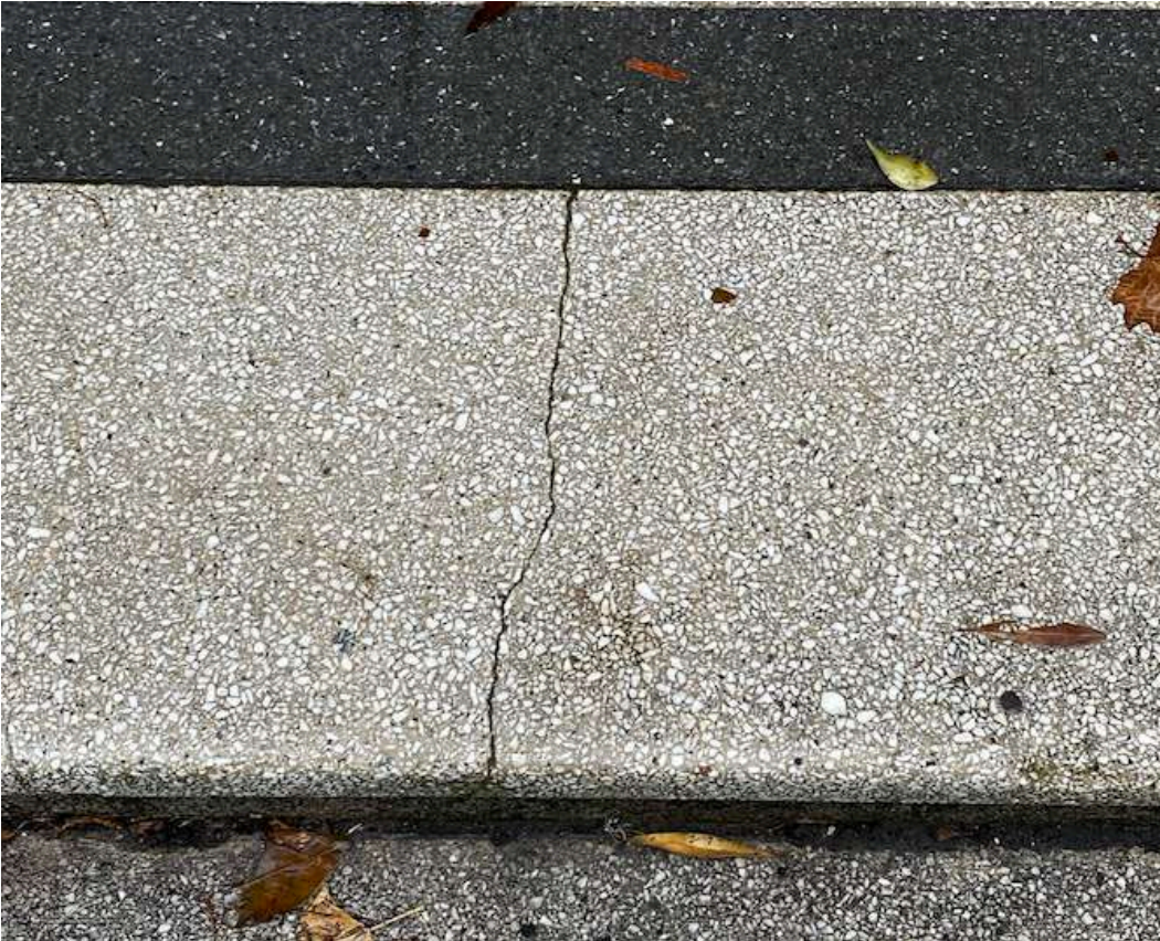
Photo. 13. The crack in the terrazzo step at the entry to the Presbytery is to be invisibly repaired by an experienced terrazzo repair contractor with a proven record of satisfactory terrazzo repairs.
