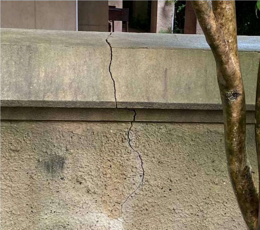
Photo. 11. Cracks in masonry are to be repaired with minimal disturbance to original heritage fabric.
