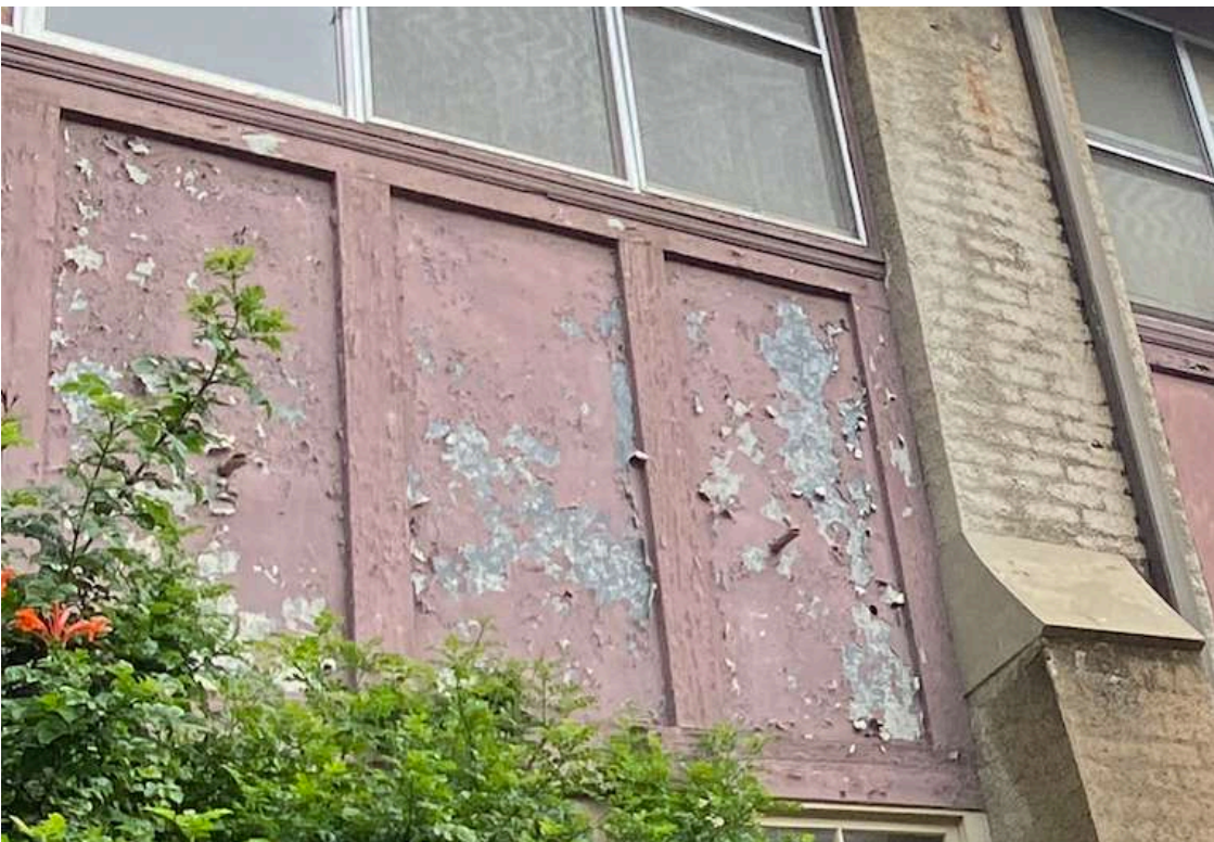
Photo. 35. All the exterior cladding and timber work is to be inspected by an experienced contractor with a proven record of satisfactory work on heritage buildings and any required repairs completed prior to properly preparing and repainting.
