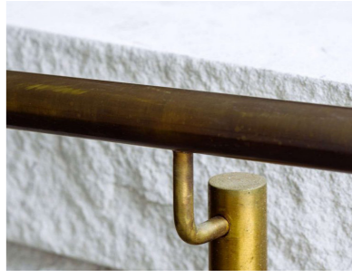
Brass Handrail to Church to AS1428
