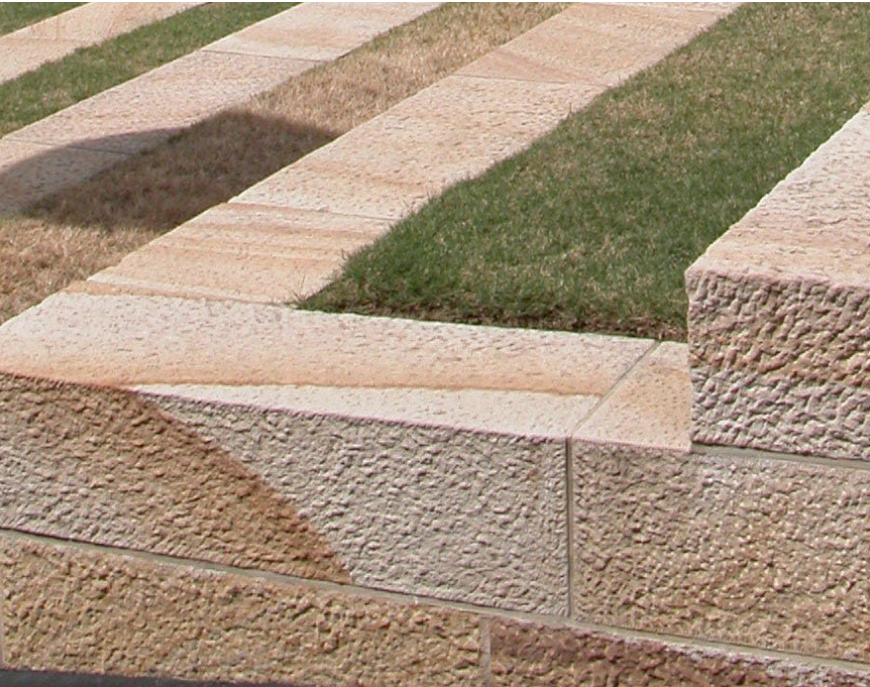
Sandstone Planter Wall
