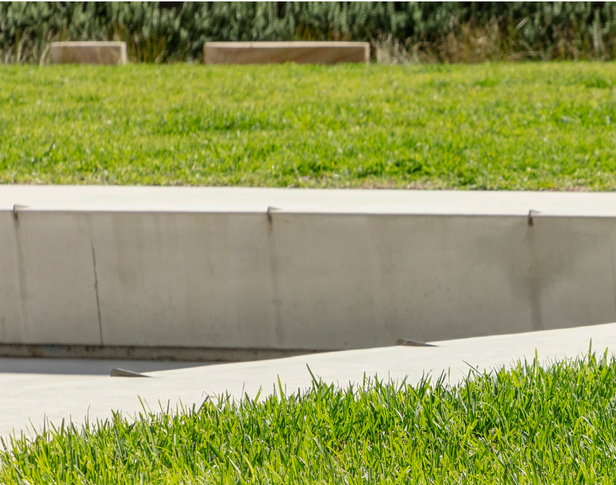
Concrete Retaining walls
