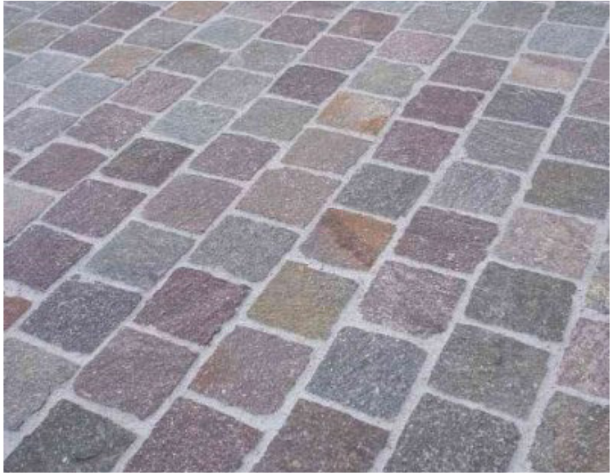
Porphyry Cobblestone Paving
