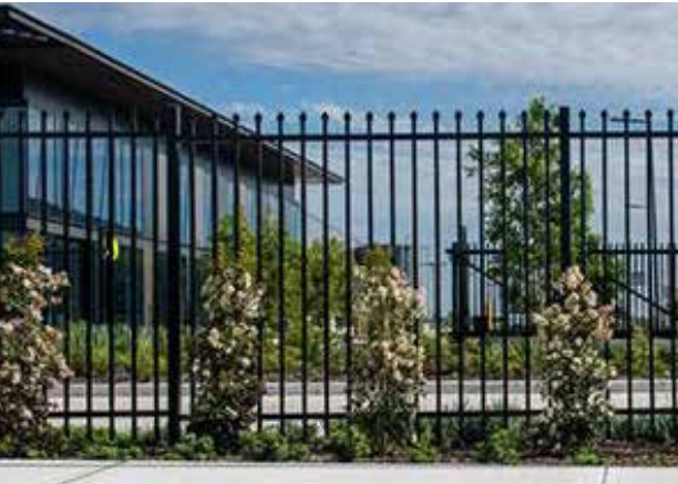
FENCE TYPE 1 EFSG-compliant boundary fence 2.15m high palisade fence
