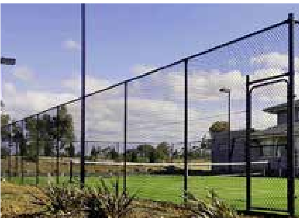
FENCE TYPE 3 2.4m high chainwire fence
