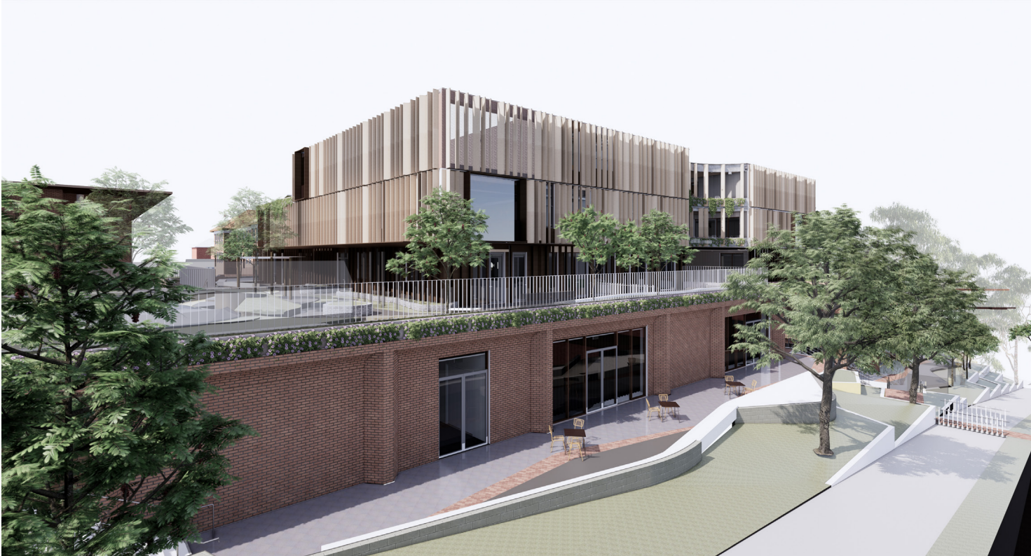
South West View - from boundary fence
