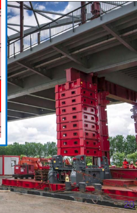
Jacking system for lowering cut bridge sections
