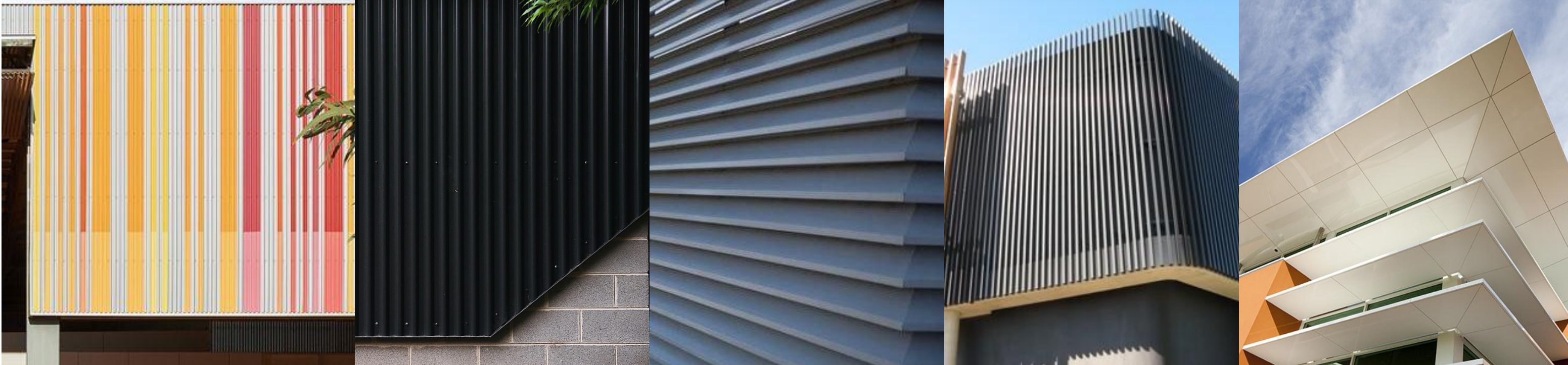
1. COLOURFUL CORRUGATE CURTAIN WALL CLADDING SYSTEM 2. SPLAYED / REDUCED CLADDING FOR REVEALS AND APERTURES 3. INTEGRATION OF SERVICES THROUGH VENTED SCREENS 4. BATTENED SCREENS FOR SUN PROTECTION, PRIVACY AND MATERIAL DEPTH 5. SUNHOODS FOR SUN AND WEATHER PROTECTION, AND TO PROVIDE DEPTH TO THE FACADE
